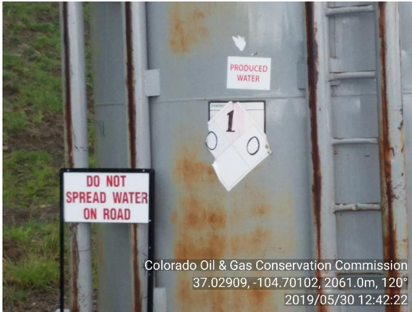
PHOTO 3: NFPA STICKER ON PRODUCED WATER TANK IS FADED AND WORN. REPLACE NFPA STICKER TO COMPLY WITH 210 SERIES RULES. CA DATE 6/30/19
