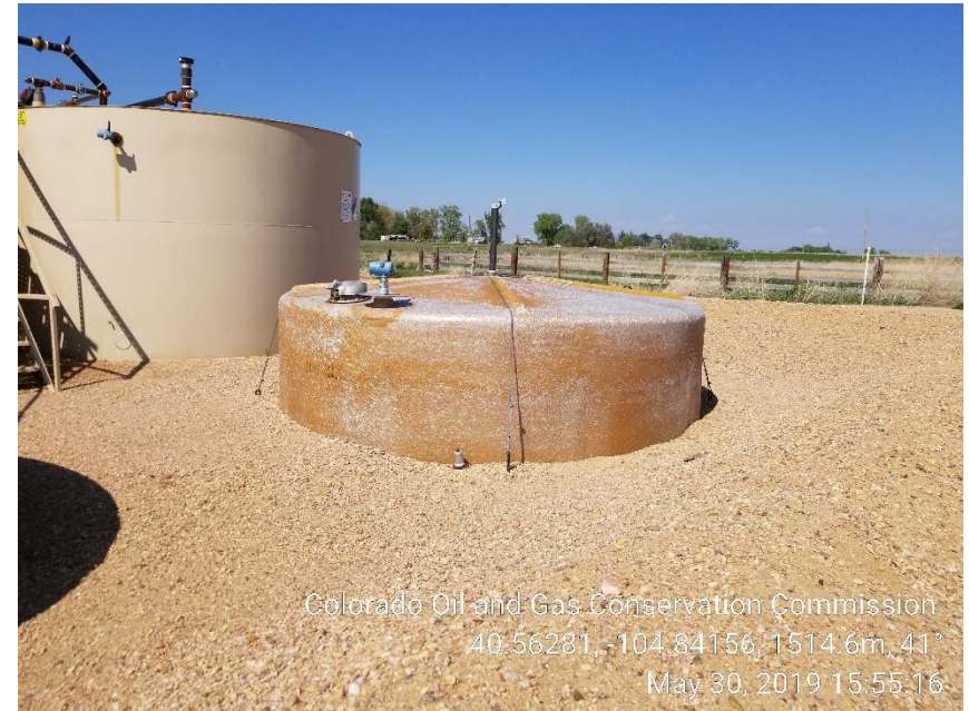
Photo 10: No NFPA placard/BBLS on produced water tank
