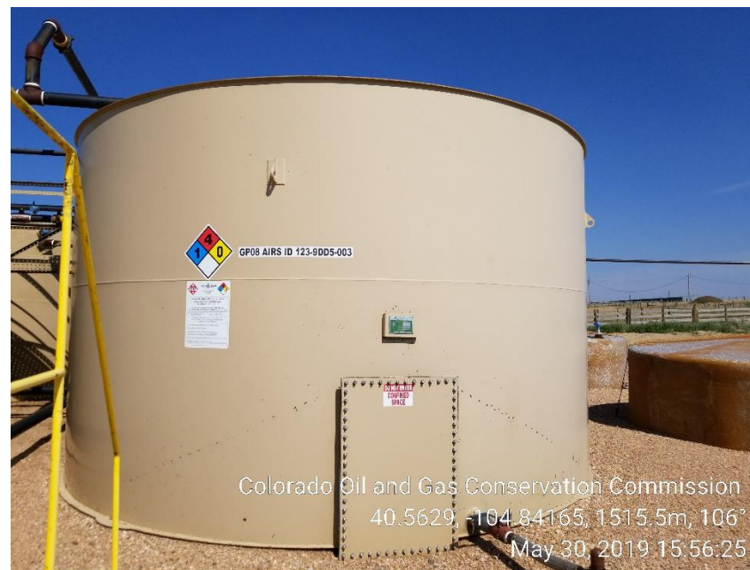
Photo 12: No labeling on tank (BBLS/contents)
