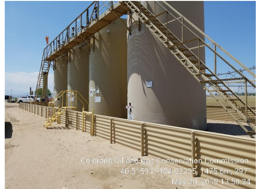
Photo 2: Tank Battery
