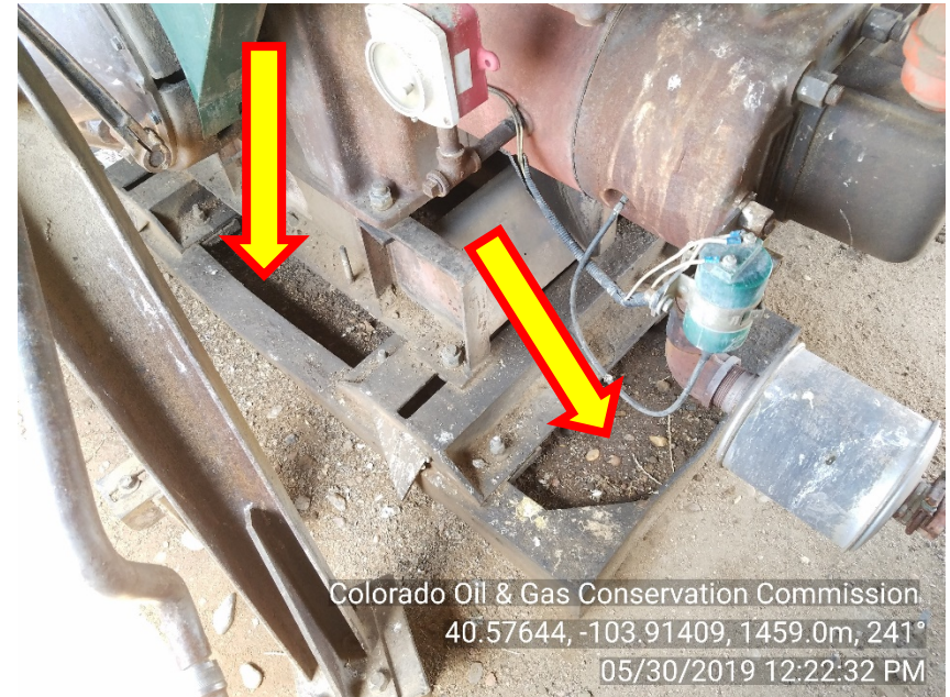
Photo #10 Nickerson 4 - Engine House Stained soil around engine base Appears NOT addressed
