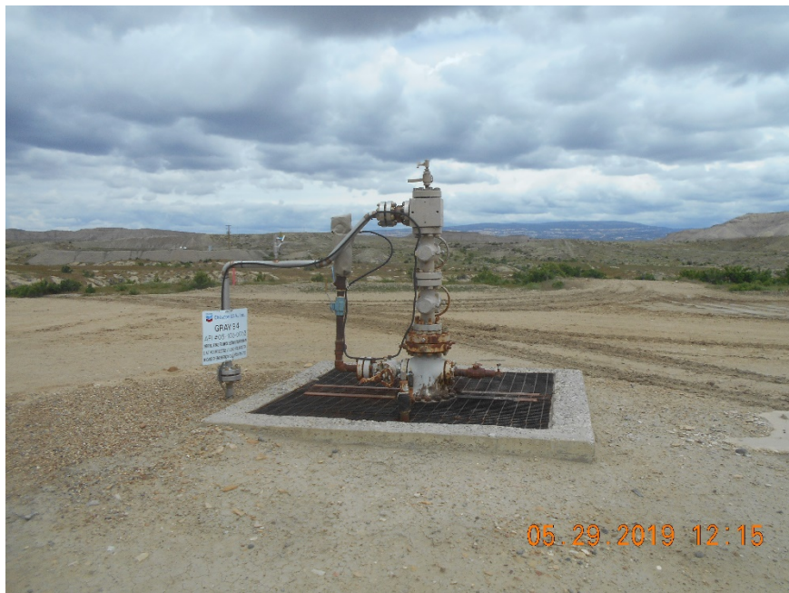
Injection wellhead
