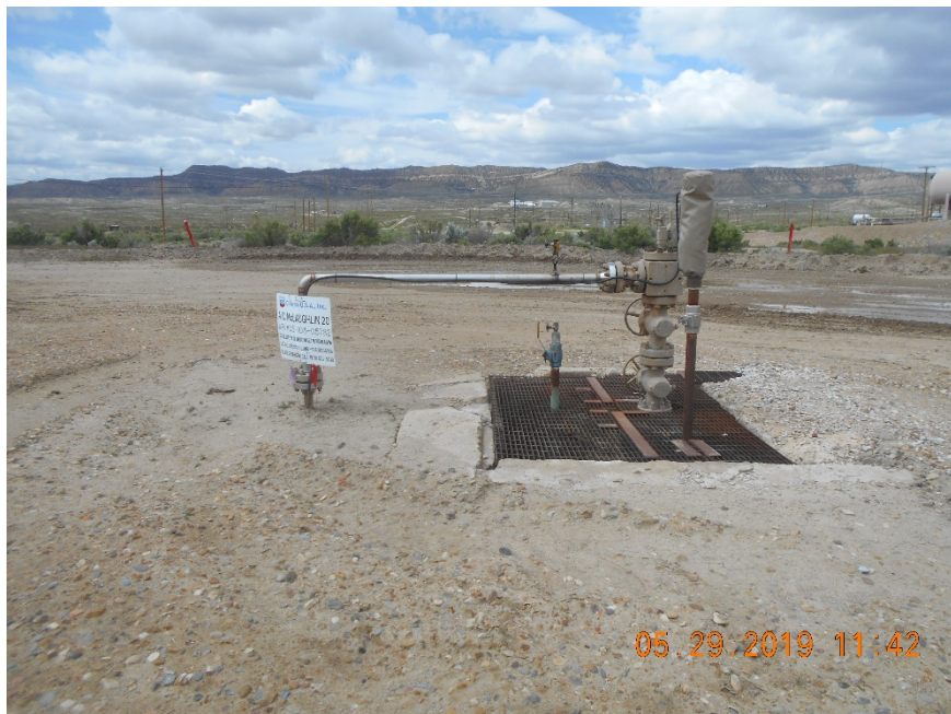
Injection wellhead
