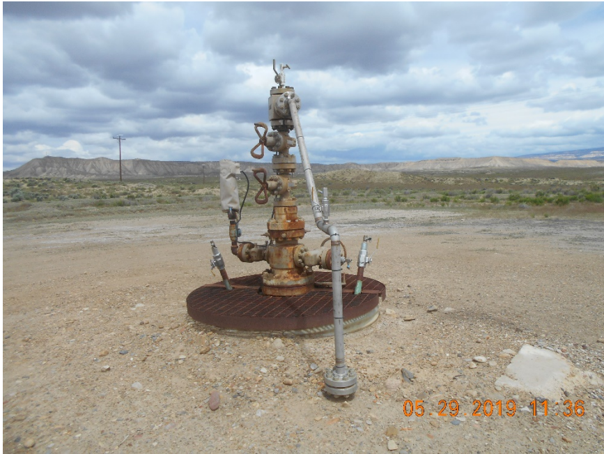
Injection wellhead
