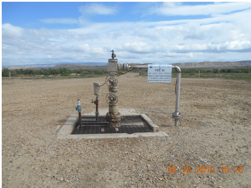
Injection wellhead
