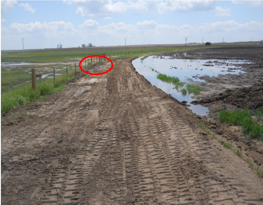
Location of breached BMP showing residual standing water and recent repair. Photo looking west. Next photo from red circled area.
