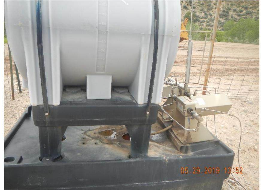
**Secondary containment under chemical containers are full and lack room to contain a possible spill.**
