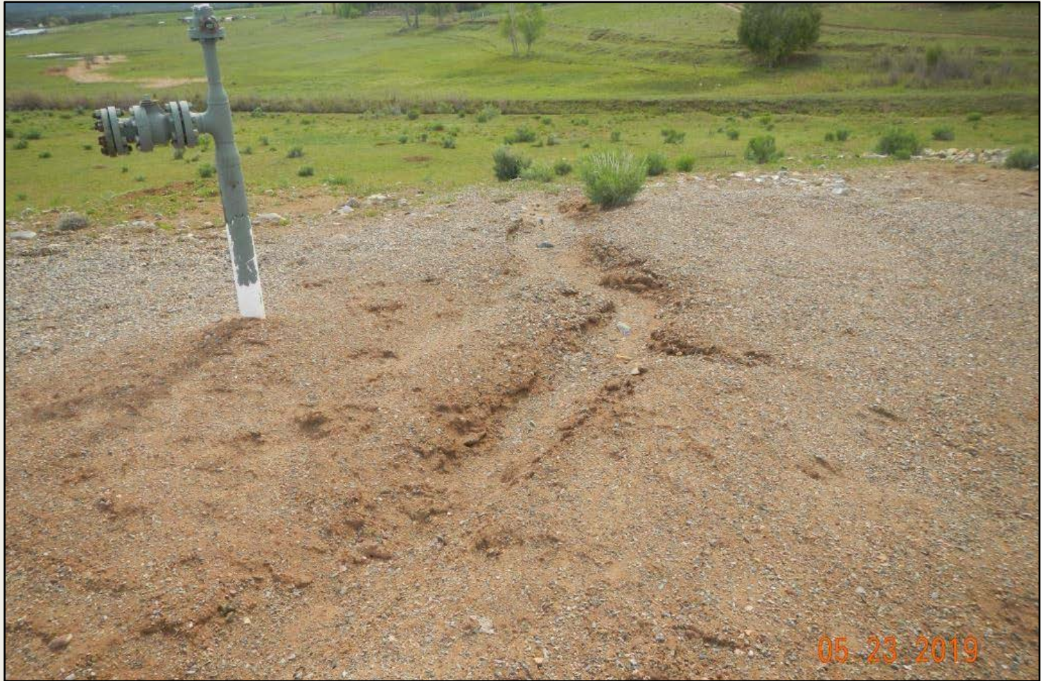
Photo 3. View of erosional channel forming within the eastern project area.
