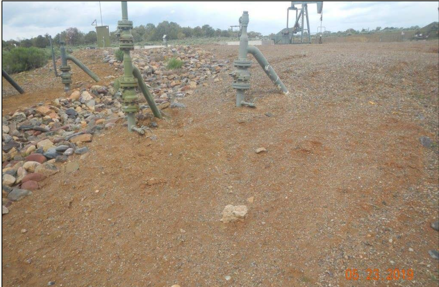
Photo 1. View of erosional scouring around cobble run-down and facilities within the southeastern project area.
