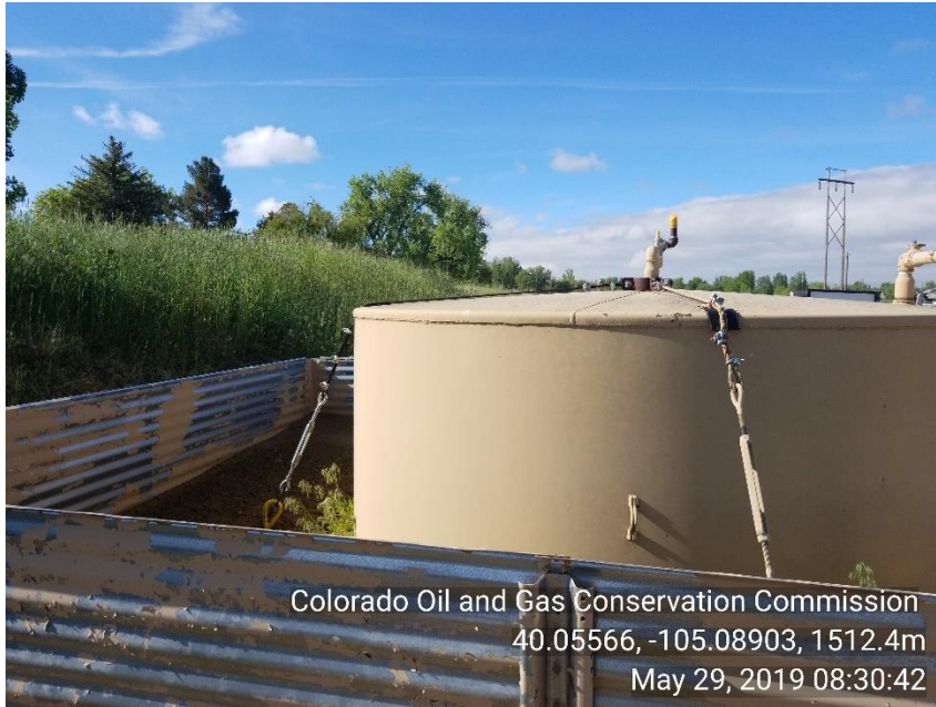
Photo 5 Anchor tie downs for condensate tank.
