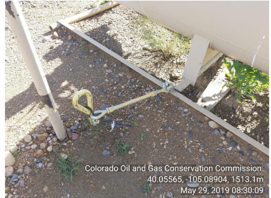
Photo 4 Anchor tie down for separator
