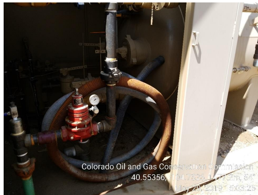
Photo 4: Tubing inside separator house.
