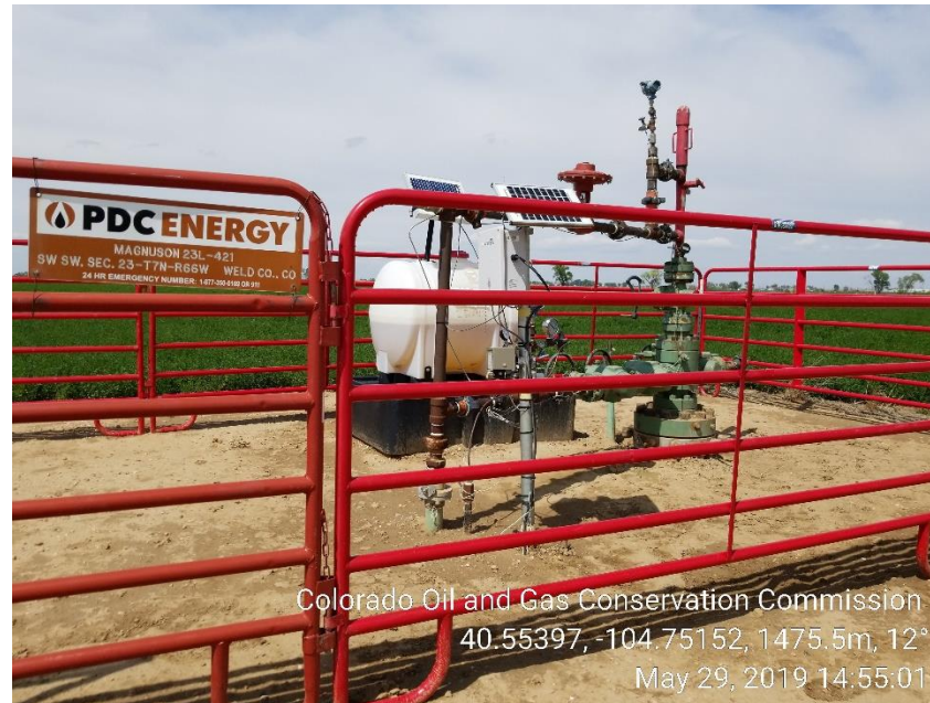
Photo 1: Wellhead w/methanol pump
