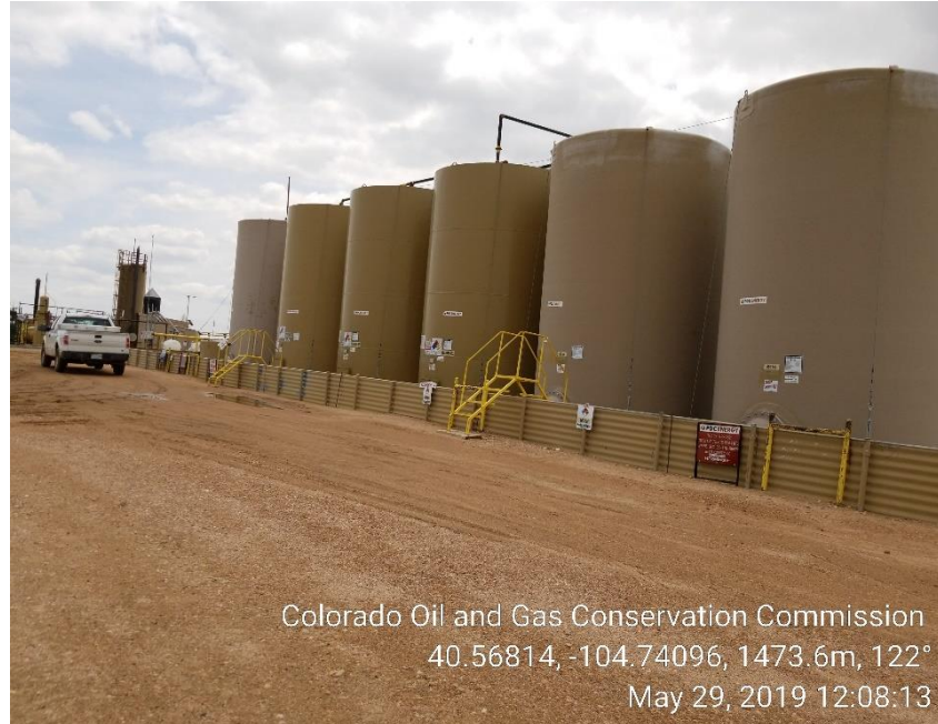
Photo 1: Tank Battery
