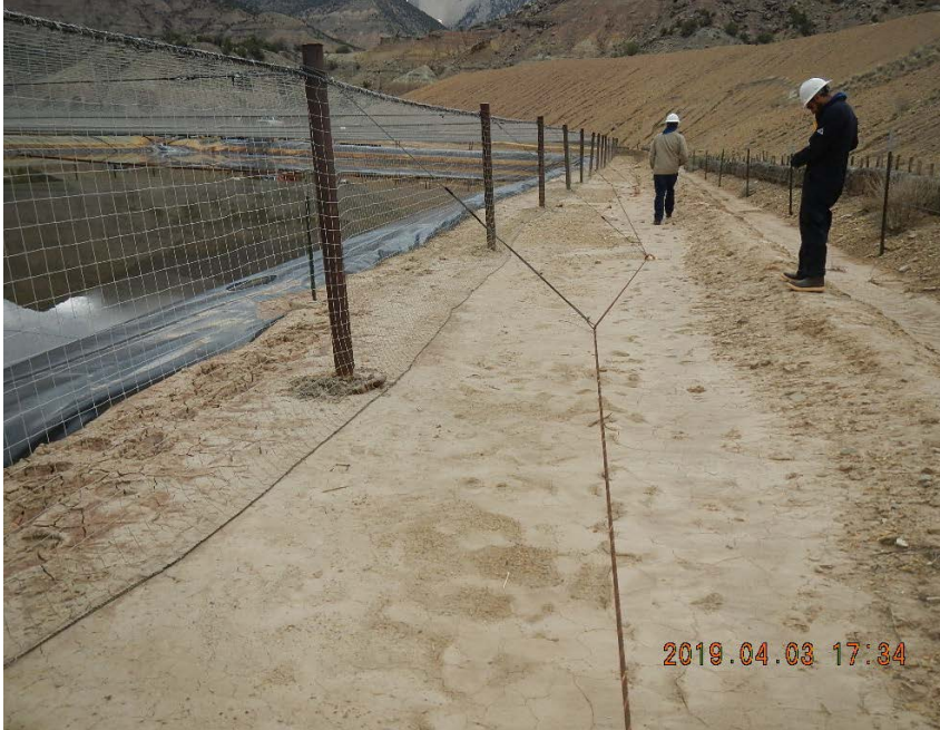
Sediment migration toward pit. Fire lane and buffer lane absent.
