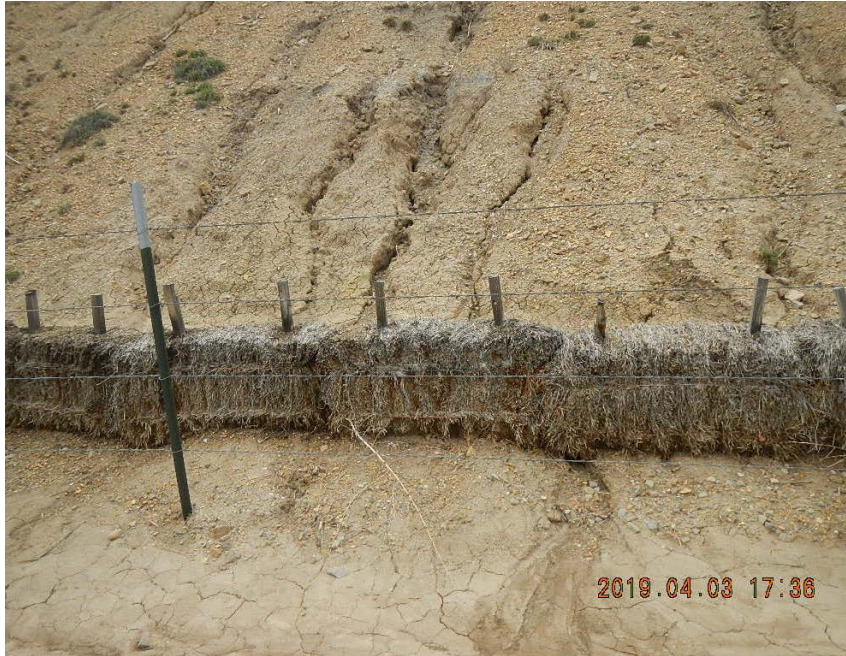
Erosional rills and failed BMPs (apparent storm water with sediment migration beneath straw bails).
