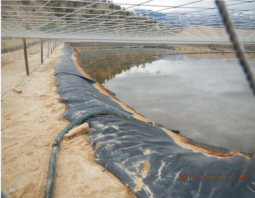
Hose and wood blocks on pit liner.
