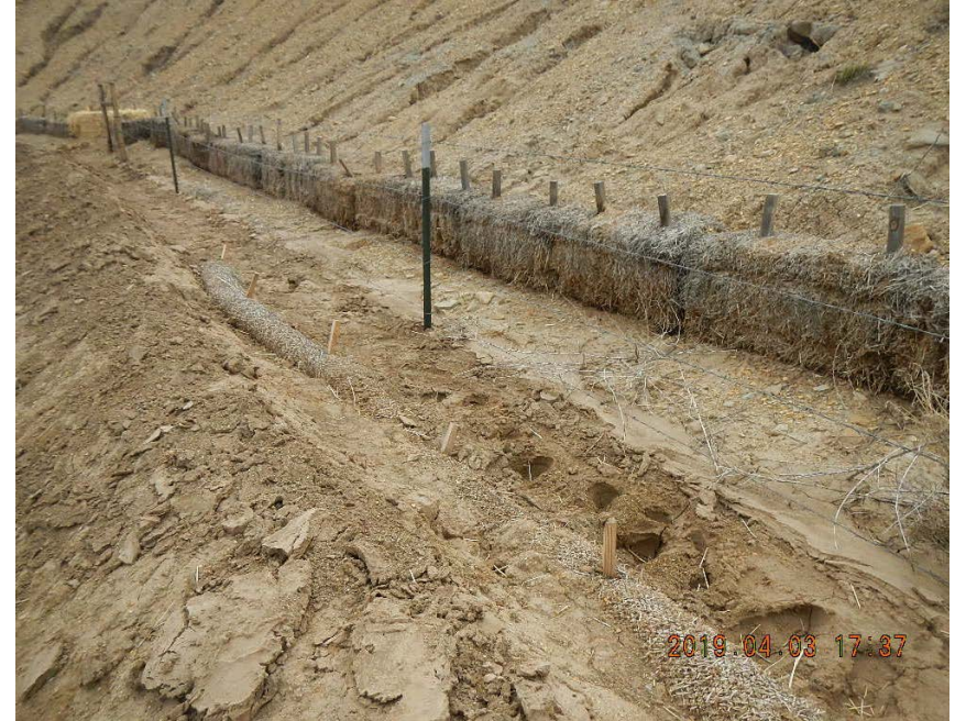
Erosional rills and evidence of livestock inside of fence.
