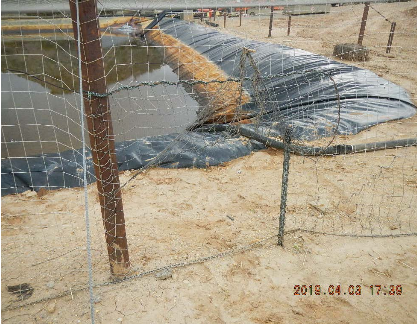
Two to three foot gap in fence/netting, hose directly on pit liner.
