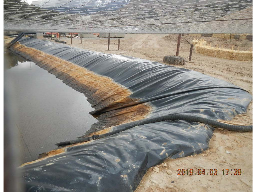
Hose directly on pit liner. Cam lock appears to have been taped.
