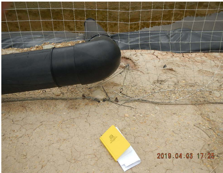
Gap in fence at pipeline penetration and sediment encroaching towards pit.
