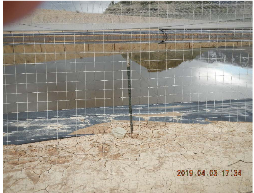
Sediment migration into pit, "T" post potentially penetrating liner near anchor trench.
