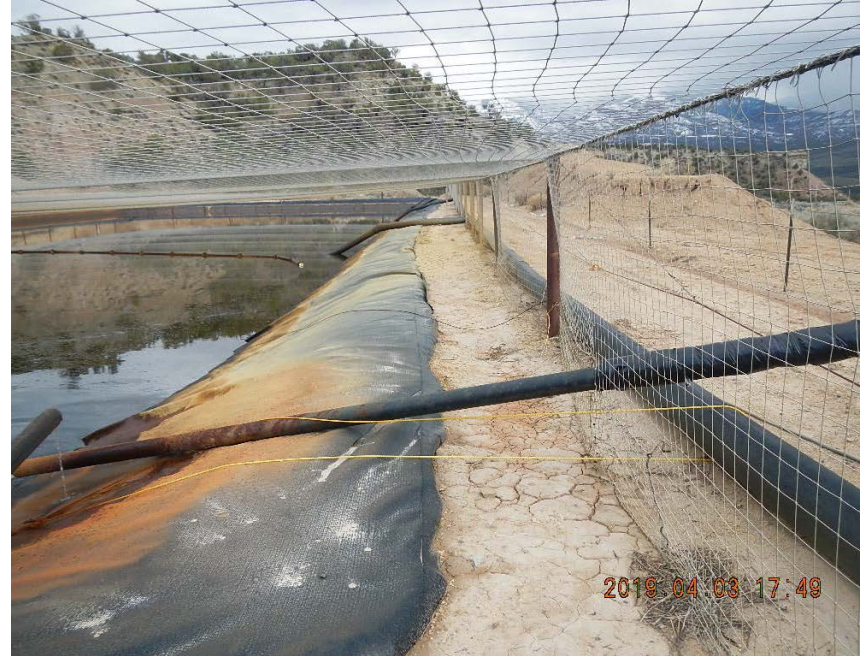
Pipe on pit liner. Yellow rope secured around poly pipe line.
