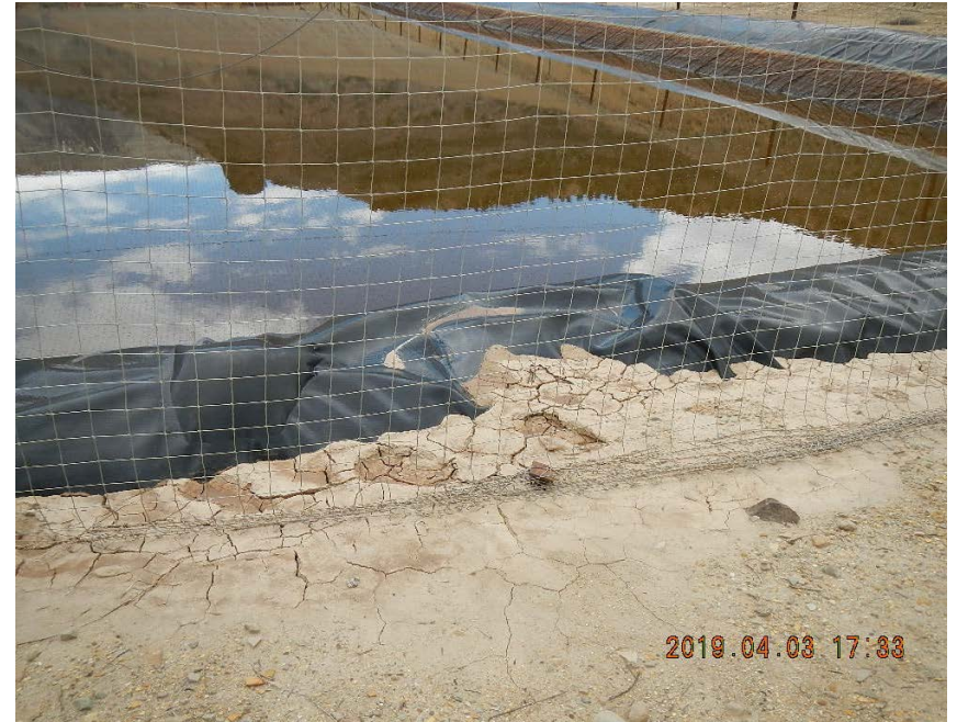
Sediment encroaching towards pit.
