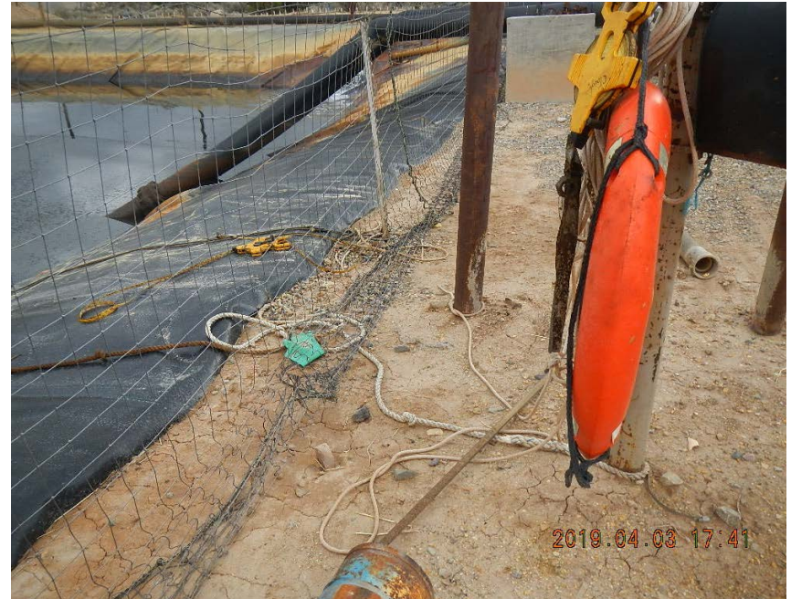
Excess equipment near manifold area. Rope safety line on liner and rescue buoy located on the outside of the netted pit.
