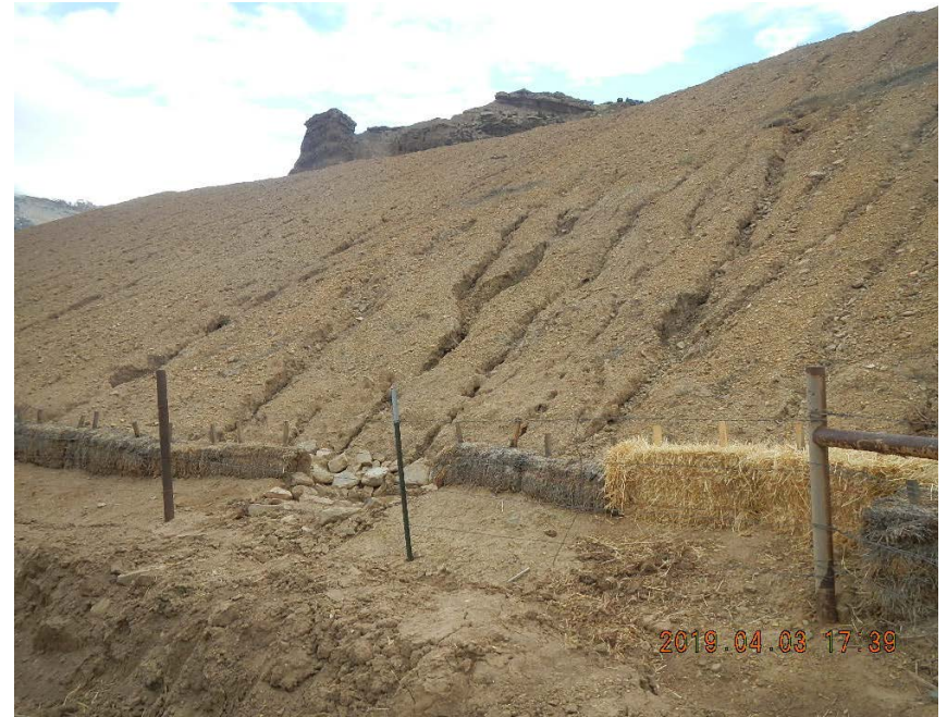
Erosional rills and recently replaced BMPs.
