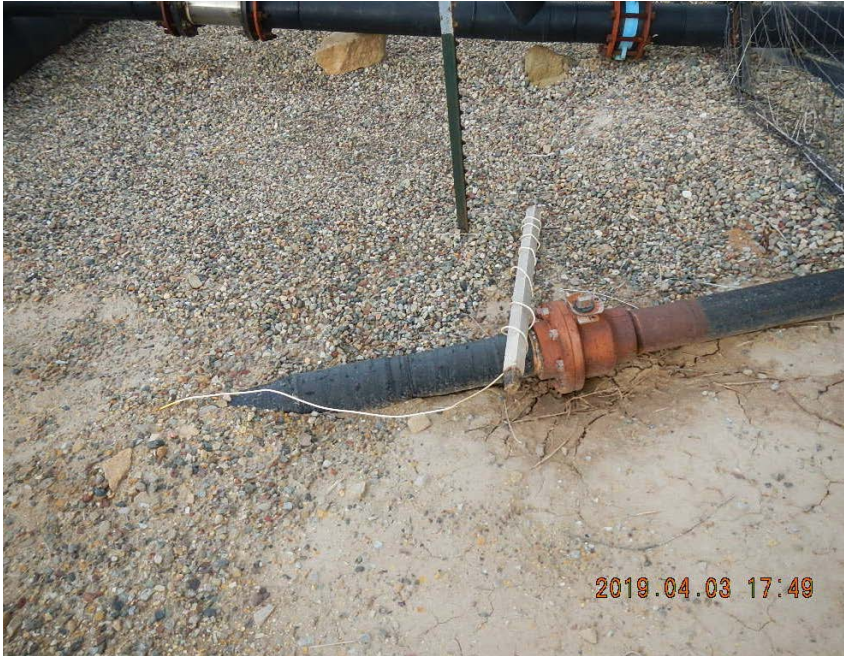
Tracer wire with stake on the ground.
