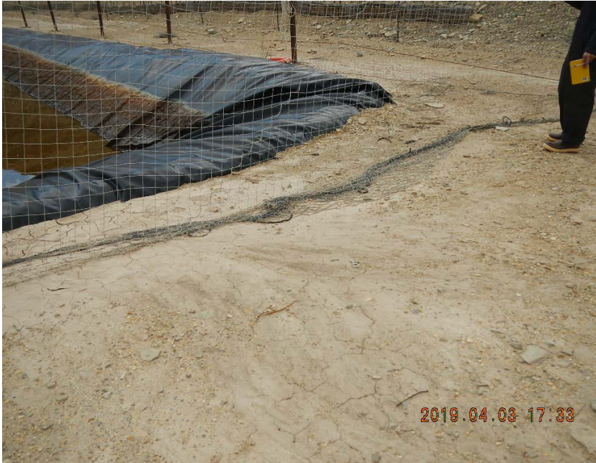
Sediment encroaching towards pit. Gaps in netting.
