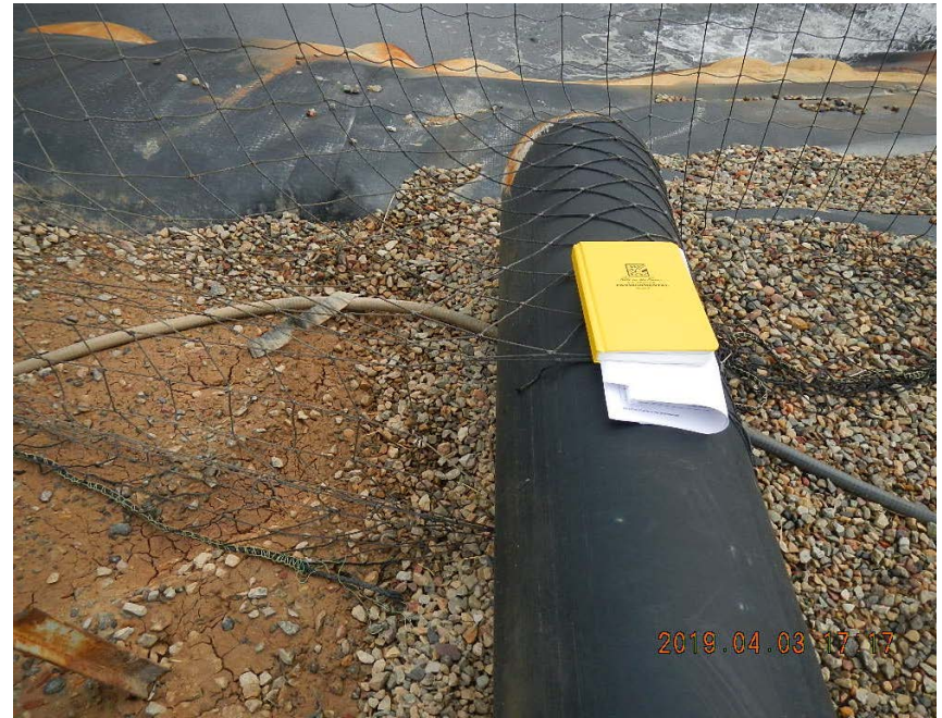
Gap in netting around pipe penetration.
