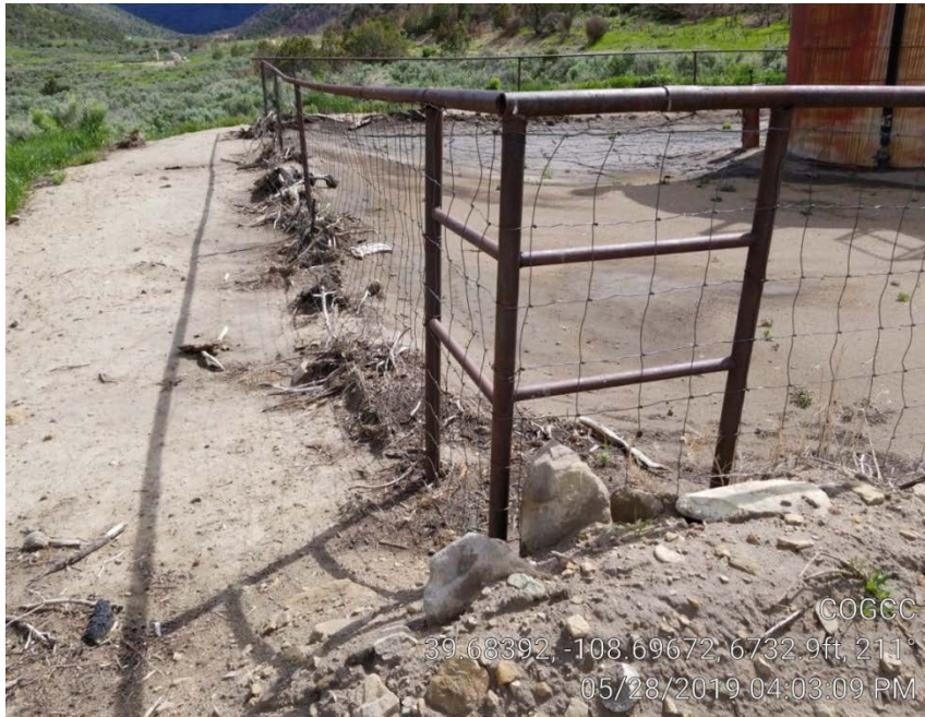
Photo 2. No berm on east side of tank battery.
