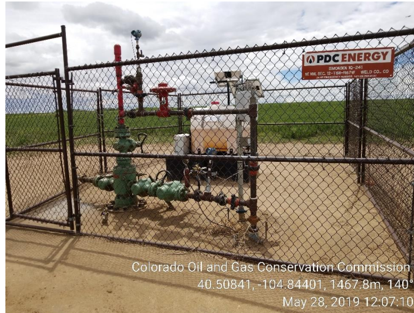
Photo 1: Wellhead w/methanol pump
