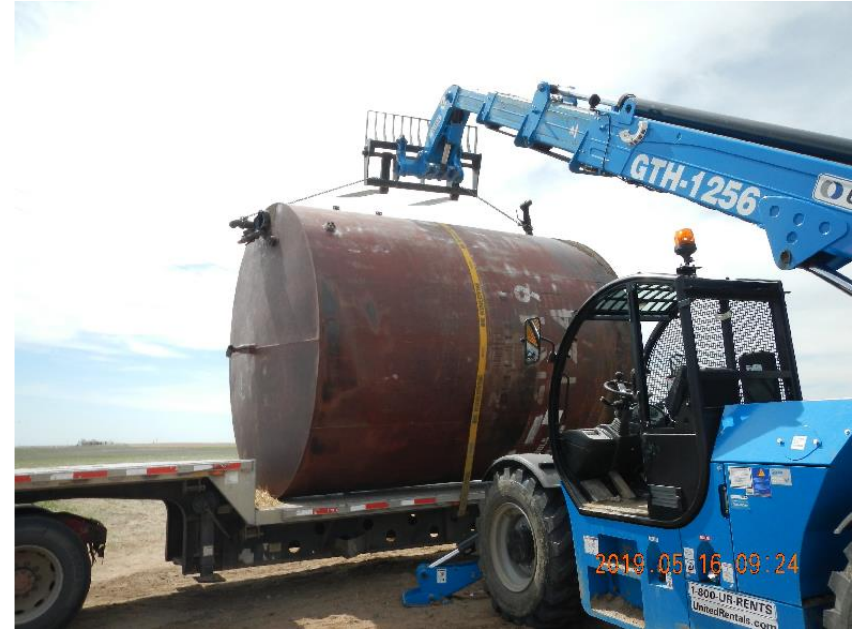
Photo 4: Water tank loaded on flatbed trailer.
