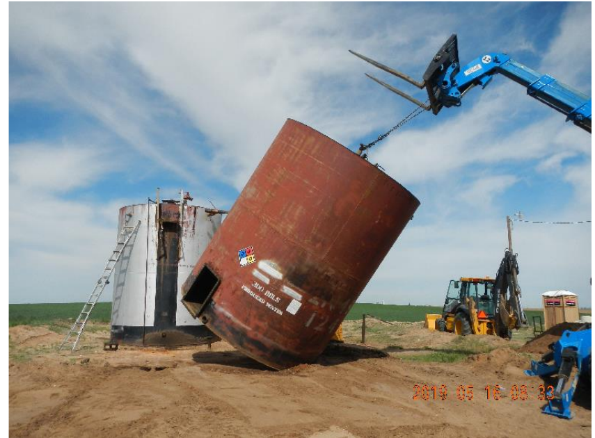
Photo 2: Laying the water tank down to be loaded.
