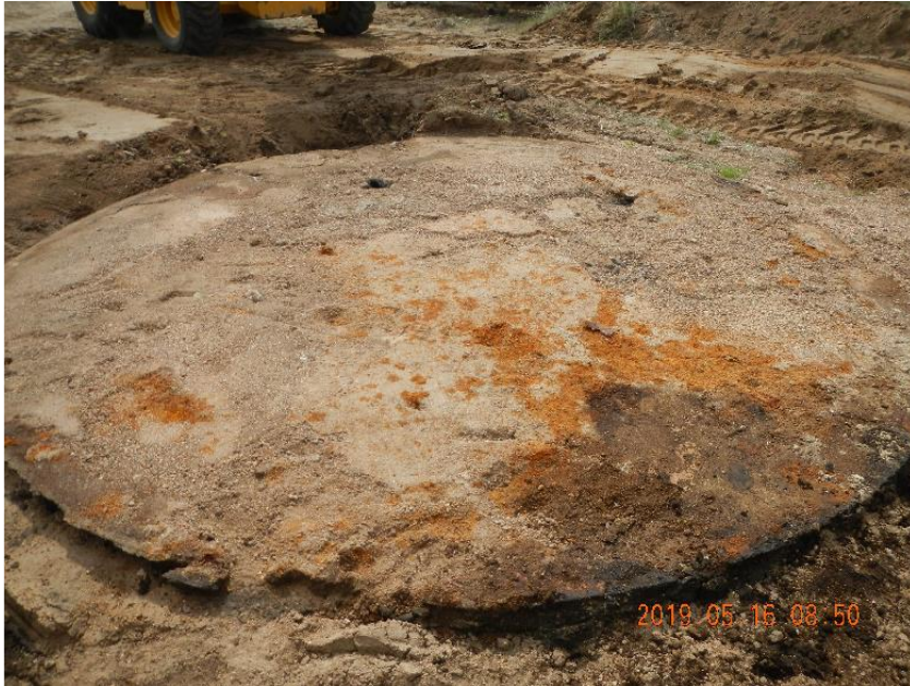
Photo 3: Soil under water tank bottom.
