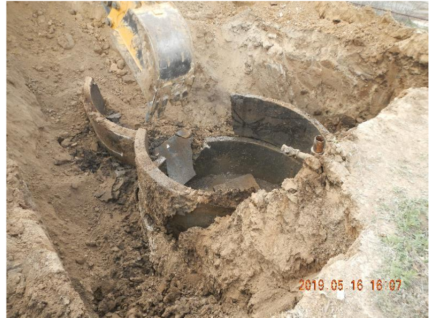
Photo 10: Breaking sump up with backhoe.
