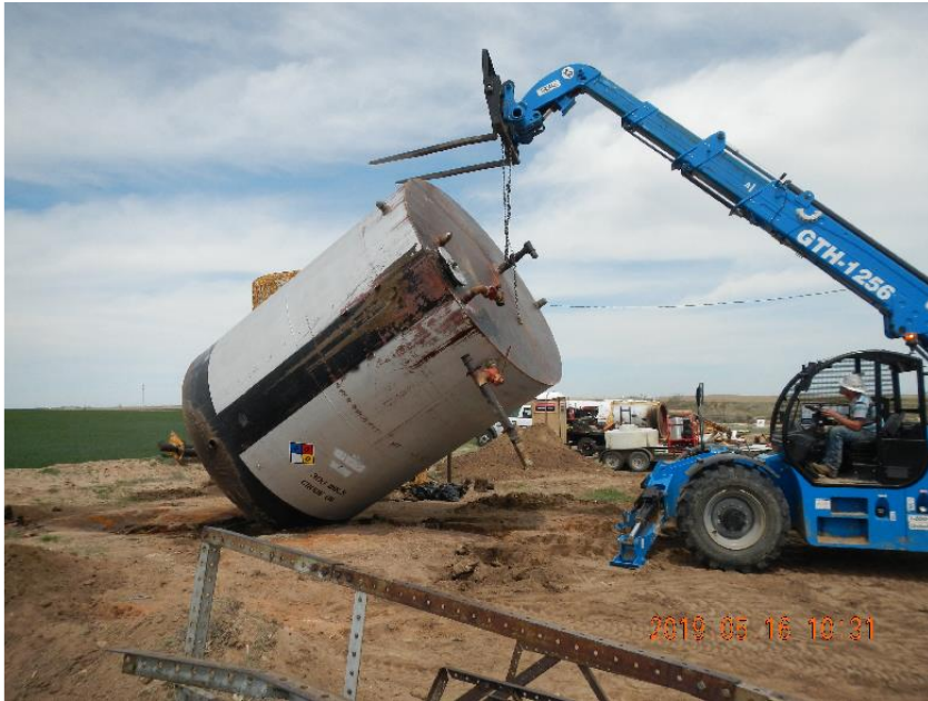
Photo 5: Laying P2 down for loading.
