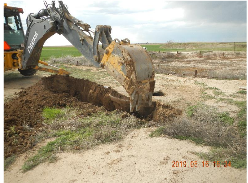
Photo 8: Excavating the concrete sump.
