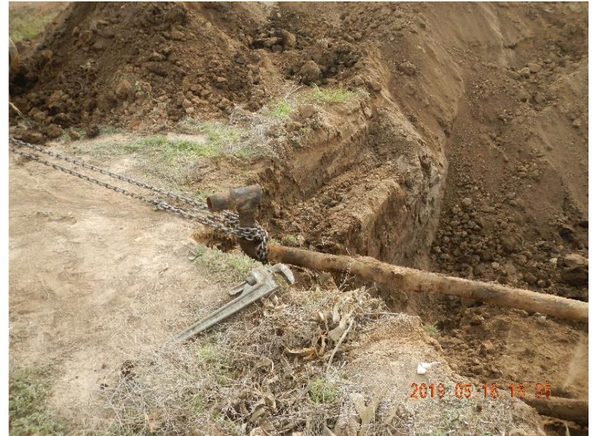
Photo 12: Pulling 3" line from sump to pit completely removing it.
