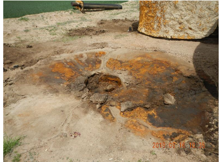
Photo 6: Soil under P2 tank bottom.
