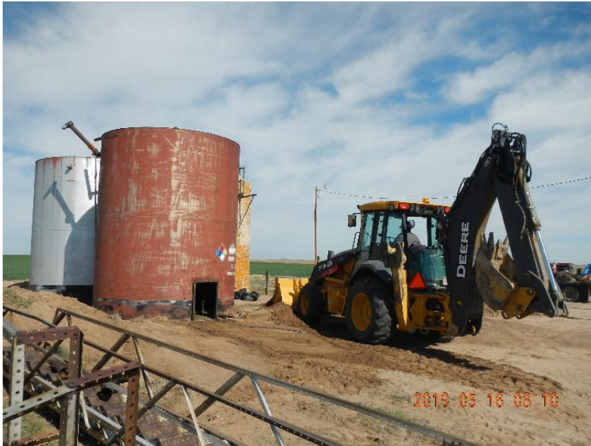
Photo 1: Opening containment berm at tank battery.
