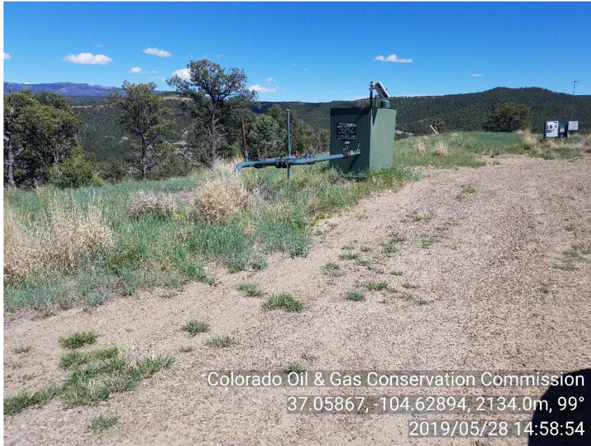
PHOTO 5: GRASS/WEEDS ON WEST SIDE OF LOCATIO AROUND METER HOUSE IS OVERGROWN. CUT OR REMOVE WEEDS IN ACCORDANCE WITH 603. SERIES RULES. CA DATE 6/28/19
