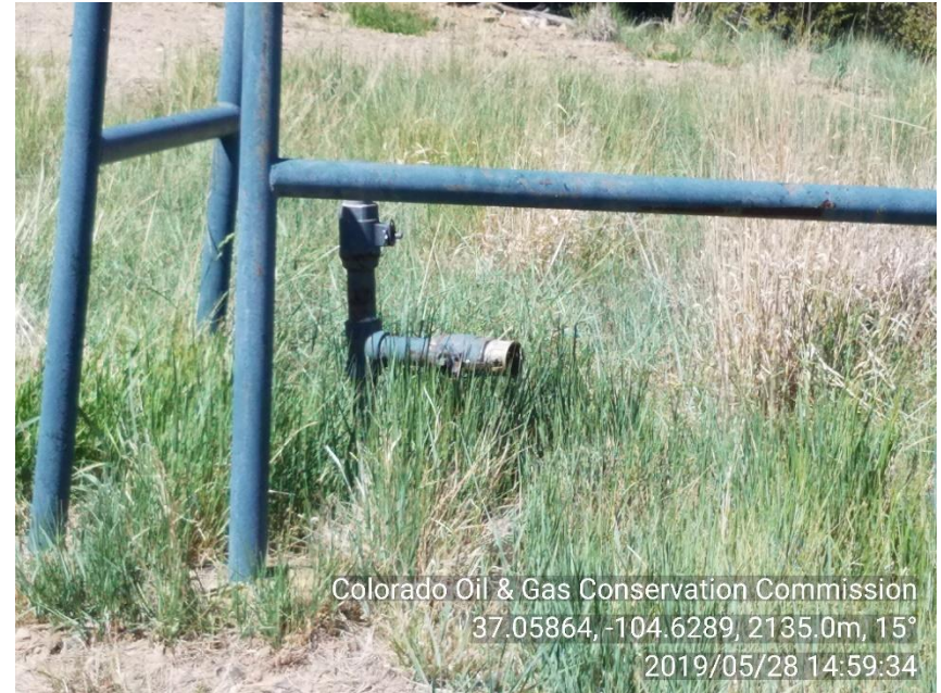
PHOTO 6: GRASS/WEEDS NEAR ENTRANCE OF LOCATIO AROUND 2" DRIP IS OVERGROWN. CUT OR REMOVE WEEDS IN ACCORDANCE WITH 603. SERIES RULES. CA DATE 6/28/19
