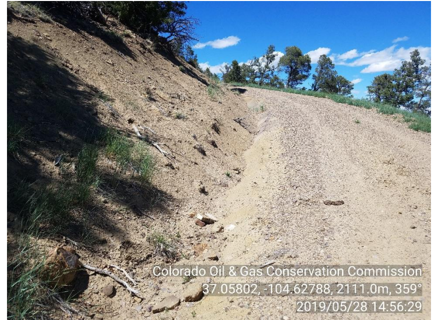
PHOTO 8: DRAINAGE DITCH ON ROW SOUTH OF LOCATION ENTRANCE HAS NO BMP'S OR BMP'S OR INADEQUATE. REPAIR OR INSTALL BMP'S TO PREVENT EROSION IN ACCORDANCE WITH 1002 SERIES RULES. CA DATE 6/28/19.
