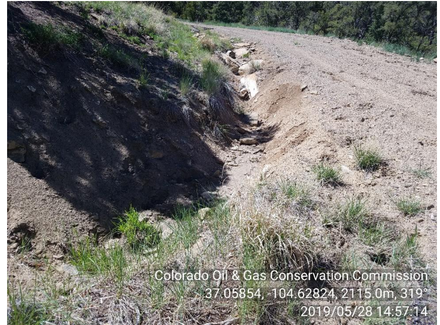
PHOTO 8: DRAINAGE DITCH ON ROW FURTHER EAST OF LOCATION ENTRANCE HAS NO BMP'S OR BMP'S OR INADEQUATE. REPAIR OR INSTALL BMP'S TO PREVENT EROSION IN ACCORDANCE WITH 1002 SERIES RULES. CA DATE 6/28/19.
