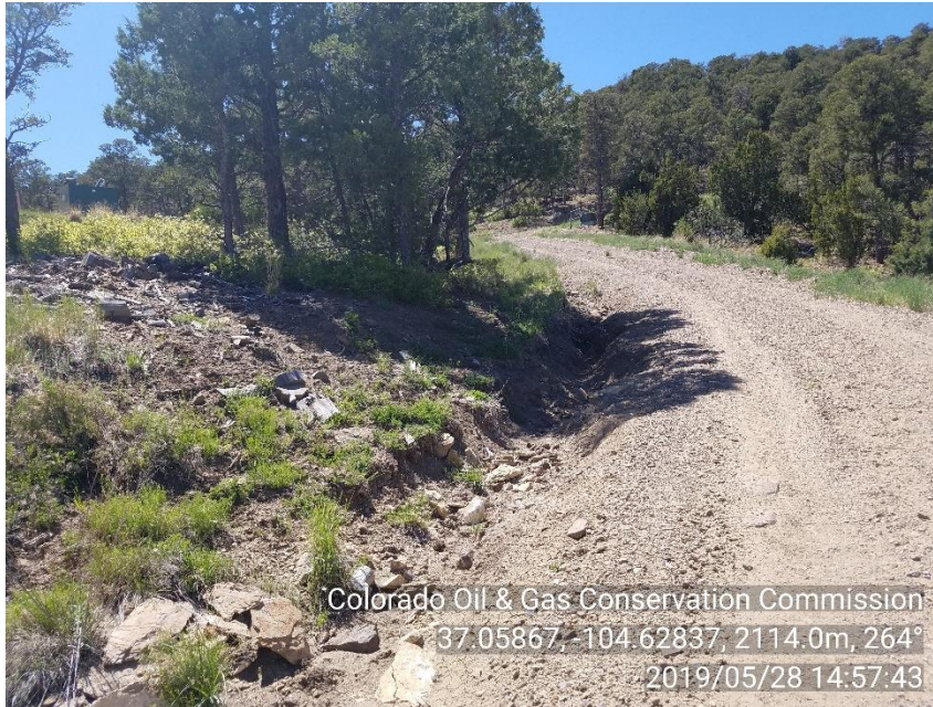
PHOTO 7: DRAINAGE DITCH ON ROW JUST EAST OF LOCATION ENTRANCE HAS NO BMP'S OR BMP'S OR INADEQUATE. REPAIR OR INSTALL BMP'S TO PREVENT EROSION IN ACCORDANCE WITH 1002 SERIES RULES. CA DATE 6/28/19.
