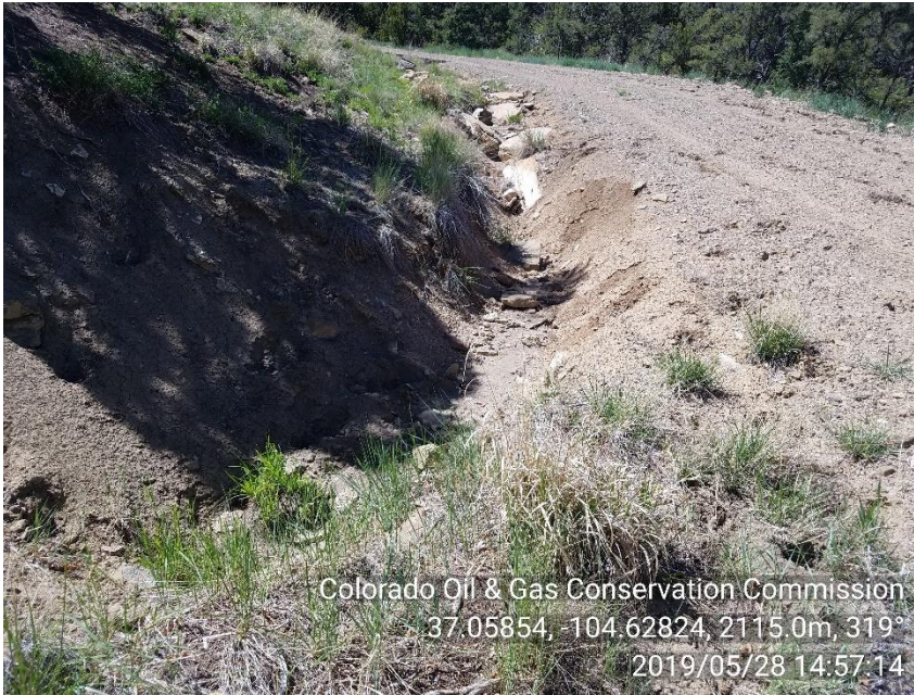
PHOTO 9: DRAINAGE DITCH ON ROW EAST/SOUTHEAST OF LOCATION ENTRANCE HAS NO BMP'S OR BMP'S OR INADEQUATE. REPAIR OR INSTALL BMP'S TO PREVENT EROSION IN ACCORDANCE WITH 1002 SERIES RULES. CA DATE 6/28/19.
