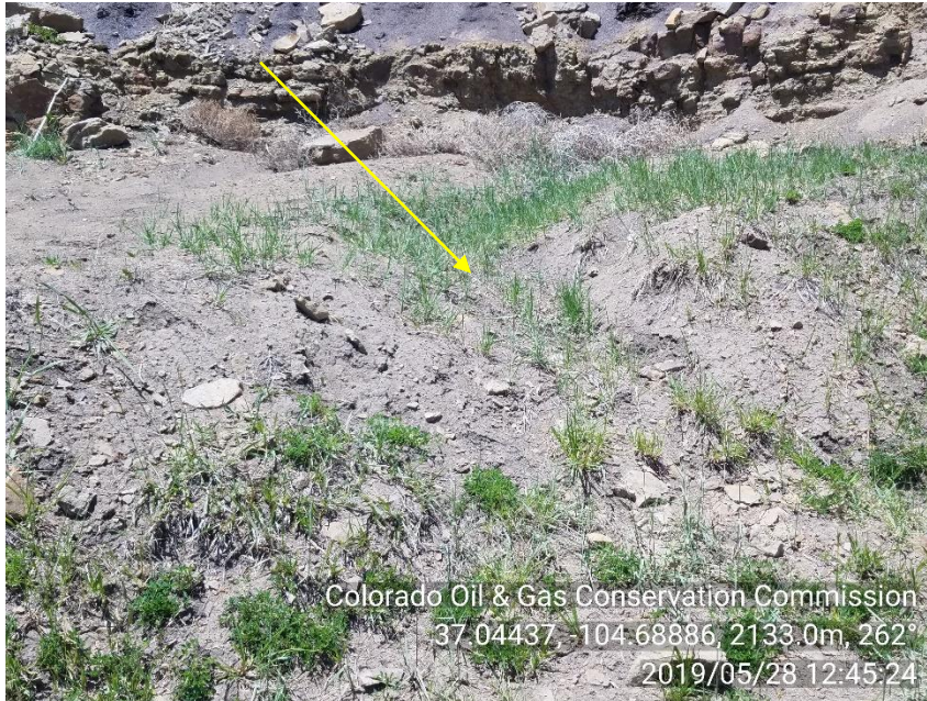
PHOTO 5: RUN ON BMP FAILURE. REPAIR RUN ON BMP IN ACCORDANCE WITH RULE 1002. CA DATE 6/28/19
