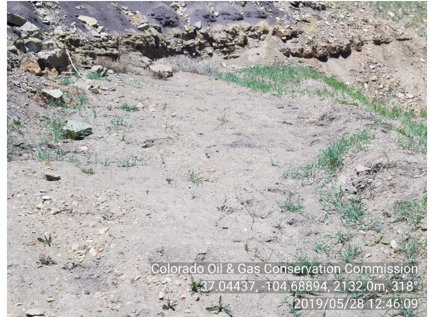
PHOTO 4: RUN ON BMP FULL WITH SEDIMENT. CLEAN SEDIMENT FROM BMP IN ACCORDANCE WITH RULE 1002. CA DATE 6//28/19.
