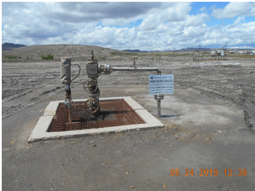
Injection wellhead
