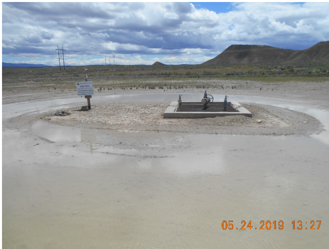
Injection wellhead – Temporarily abandoned
