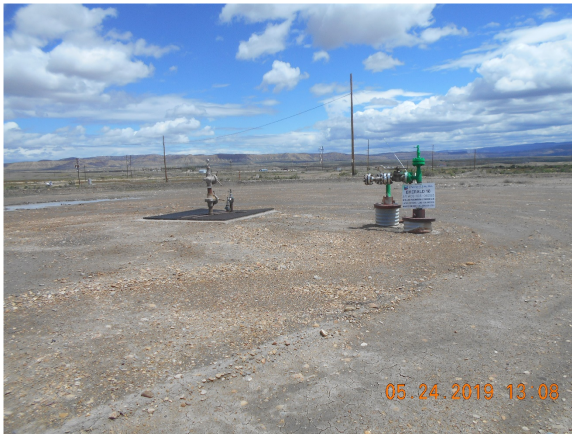
Injection wellhead – Temporarily abandoned
