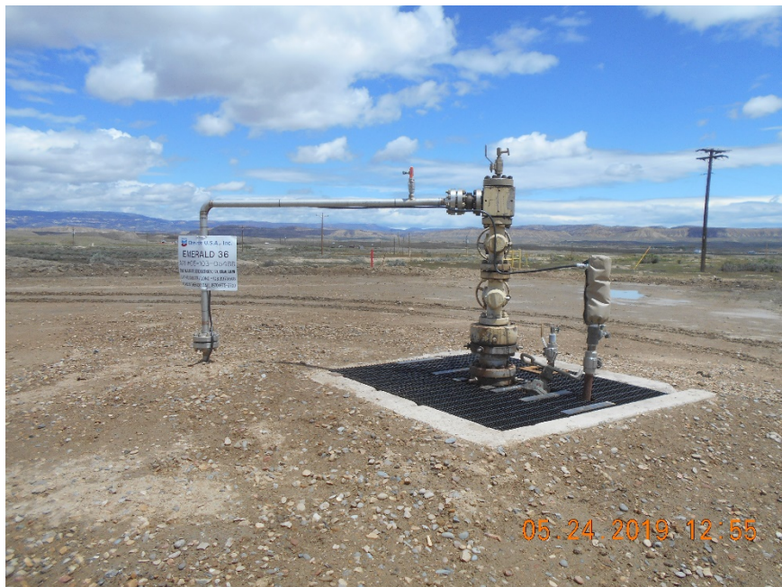
Injection wellhead
