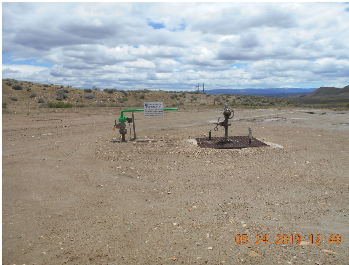
Injection wellhead – Temporarily abandoned
