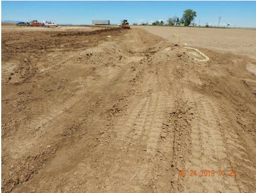
Photo 1. Photo taken from the southeastern location, facing North. Ditch and berm BMP has been installed around the entire perimeter of the location in conjunction with other BMPs (i.e., sediment traps). Operator plans to install a larger permanent sediment trap prior to drilling operations.
