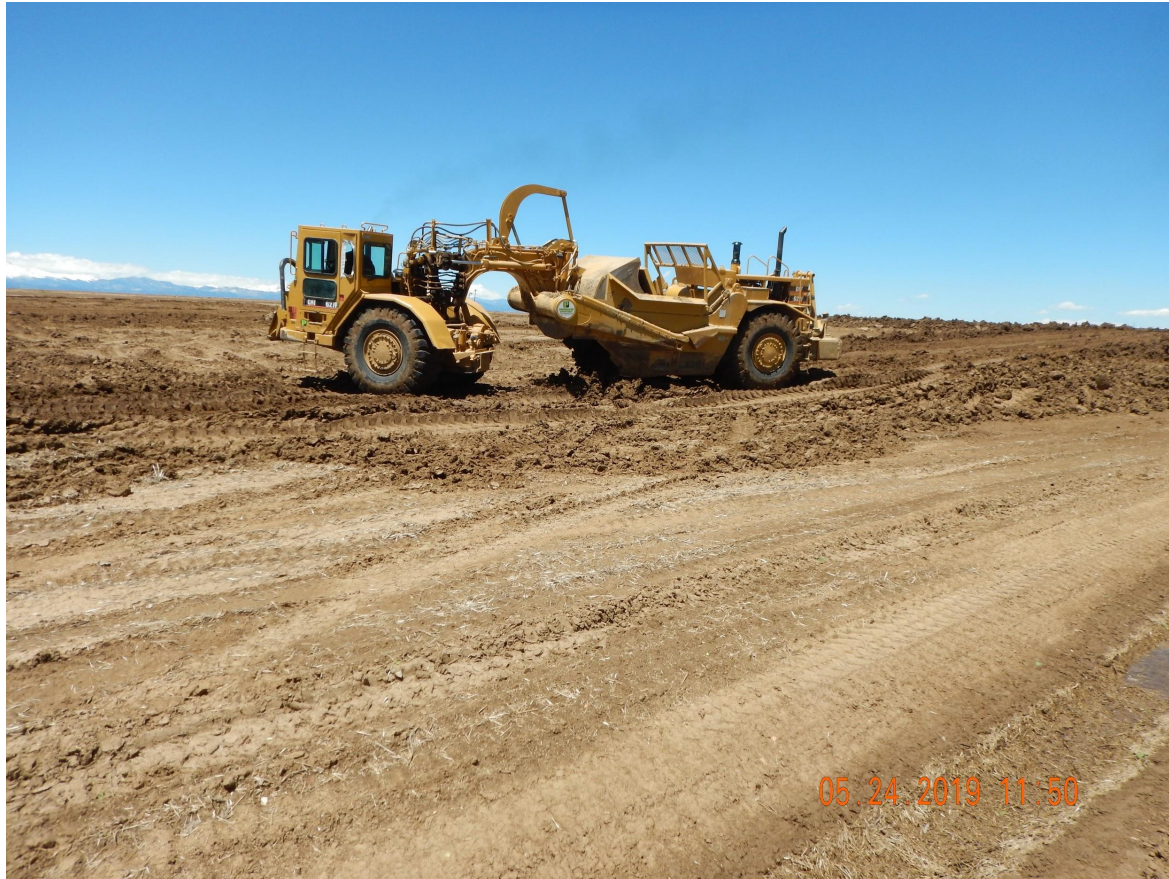
Photo 7. Photo taken from the second topsoil stockpile, facing Northwest. Topsoil salvage operations were in process during the time of this inspection.
