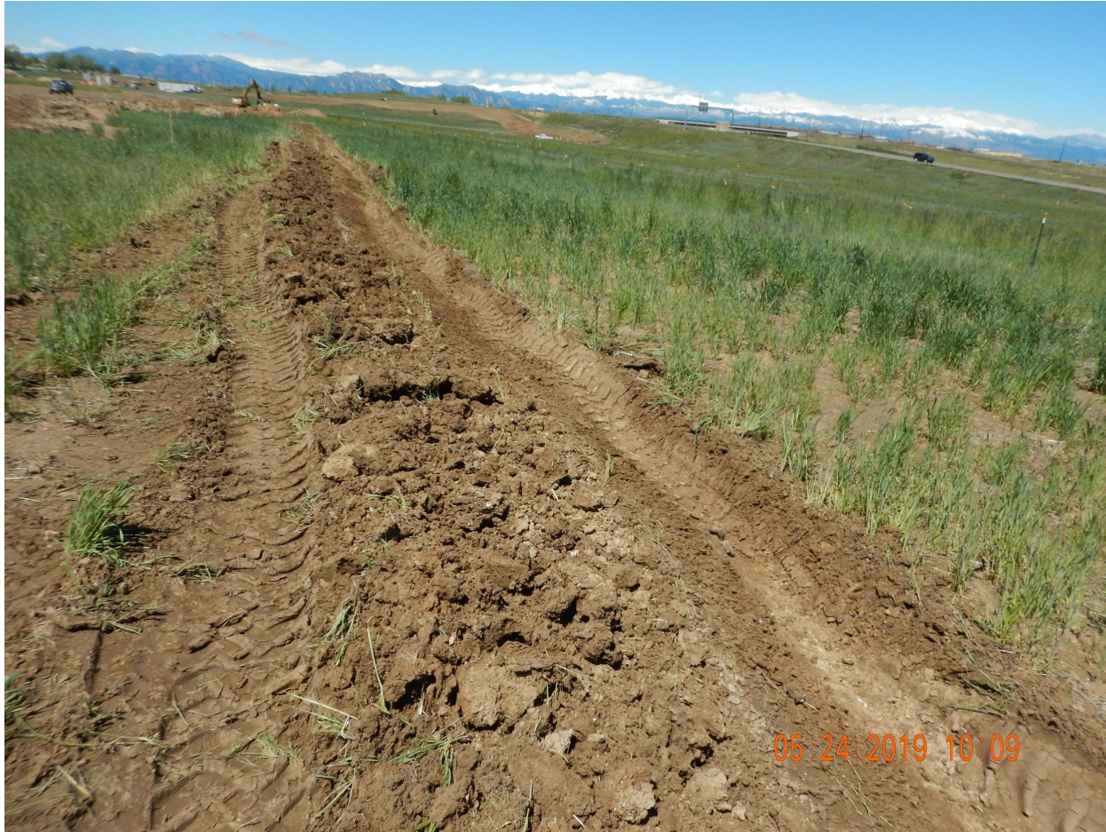
Photo 1. Photo taken from the southwestern perimeter of the location, facing West. A berm BMP has been installed around the perimeter of the location but it has not been installed with good engineering practices. The berm BMP has not been stabilized. Note: Other disturbances in the foreground are not associated with oil and gas operations.
