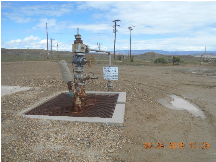
Injection wellhead
