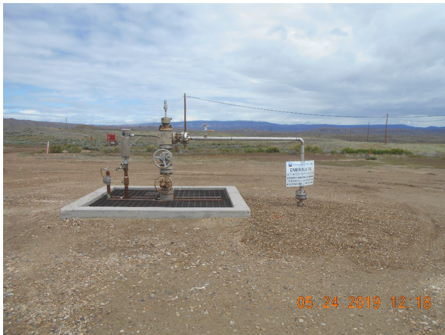
Injection wellhead
