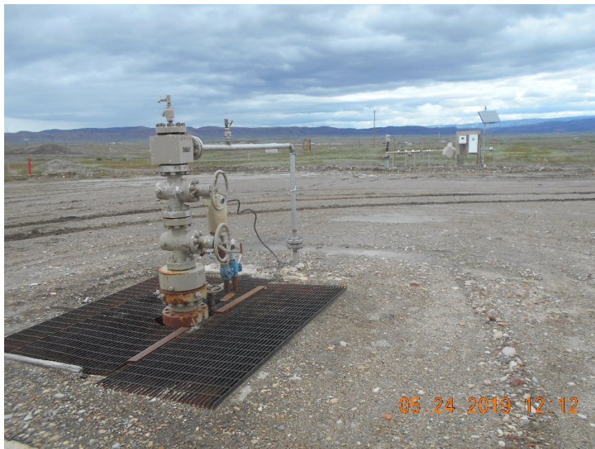
Injection wellhead
