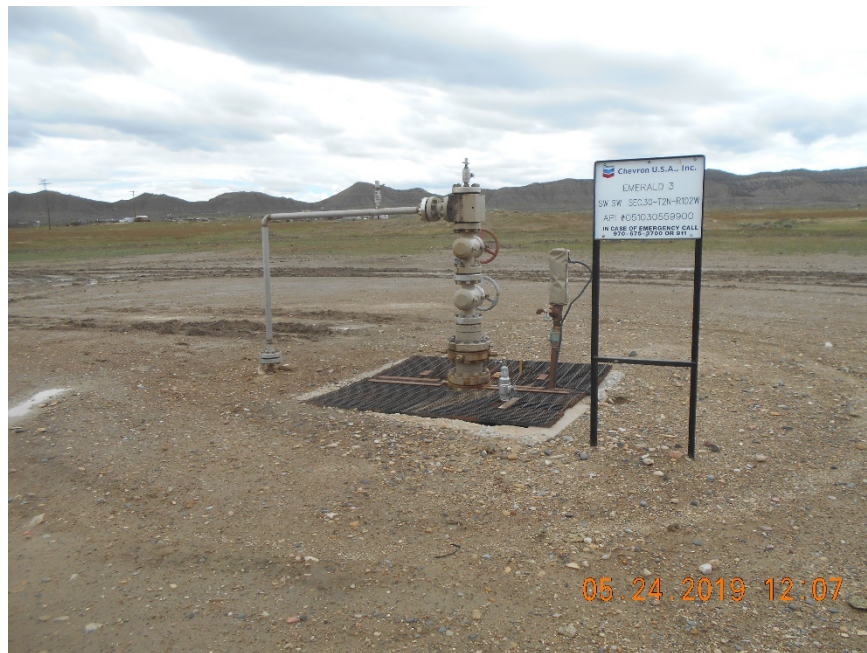
Injection wellhead
