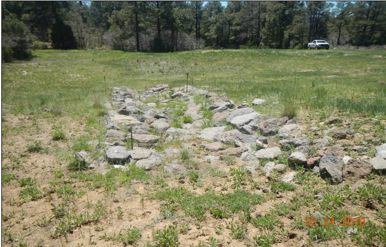
Photo 3. Facing south at the location. Rip/rap is placed in drainage channel.
