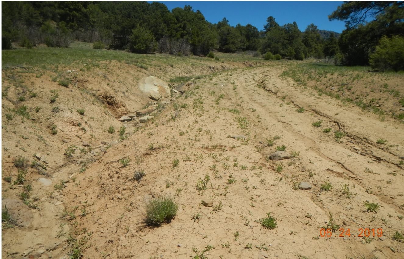
Photo 1. There is erosion issues along the main road to the location. Lat/Long:37.02250,-104.48266. The road was widened during operations.
