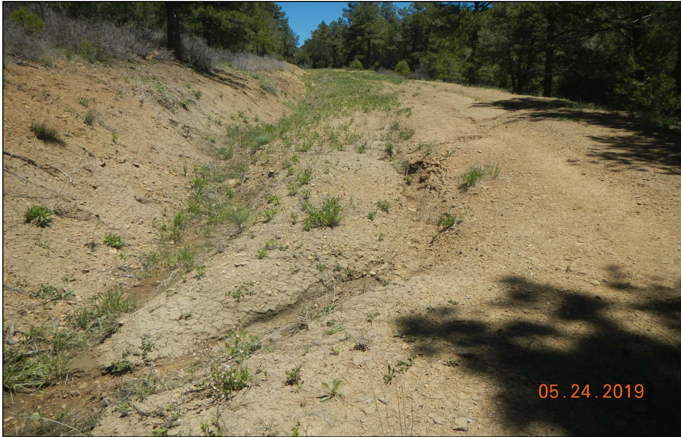
Photo 3. There is erosion issues along the road traveling toward the location.
