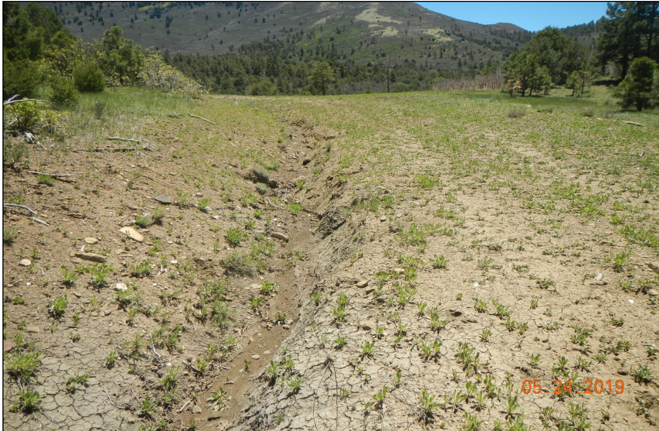
Photo 5. There is an erosion channel near the location along the road..
