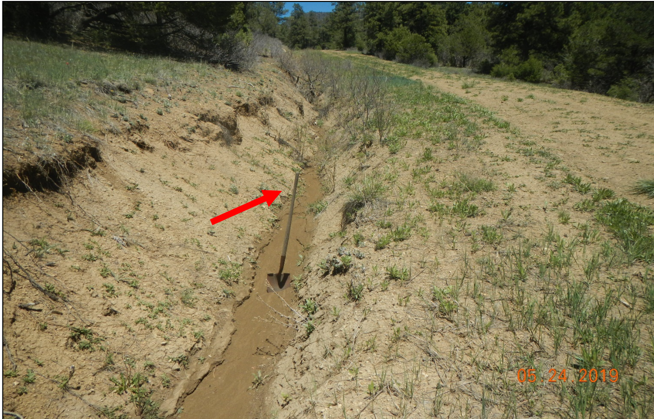
Photo 2. There is a deep channel that developed along the side of road. Arrow points to 4.5 ft. shovel to show depth.
