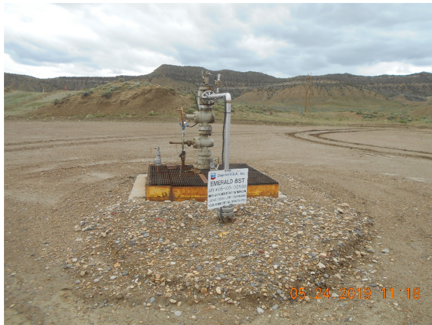
Injection wellhead
