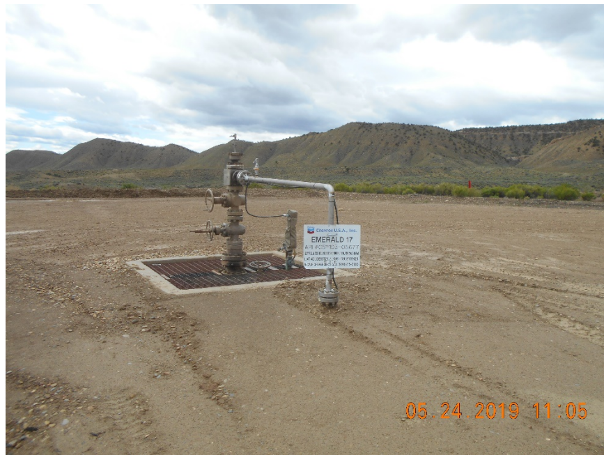
Injection wellhead
