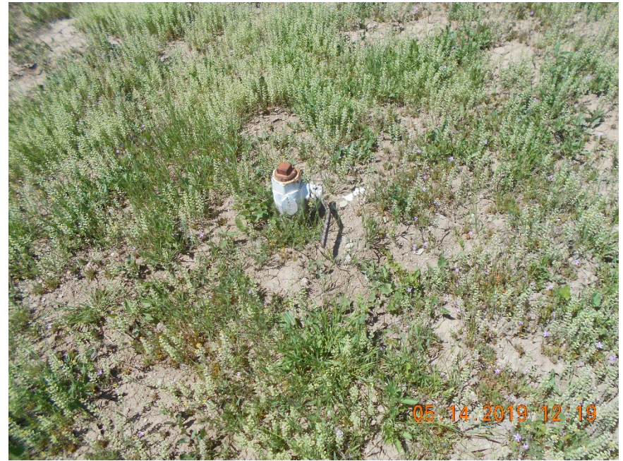
Unused riser E. of equipment
