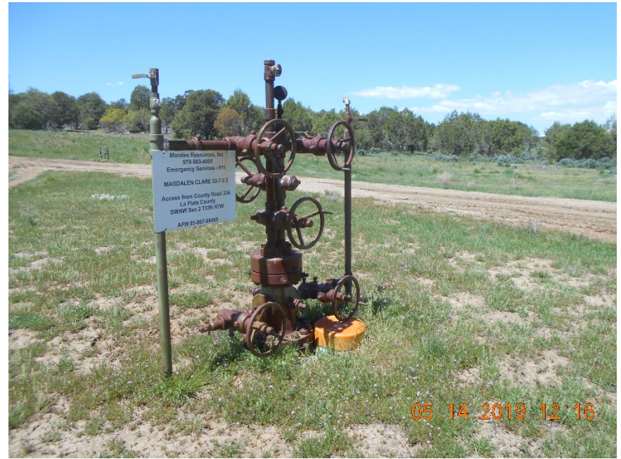
Wellhead with sign
