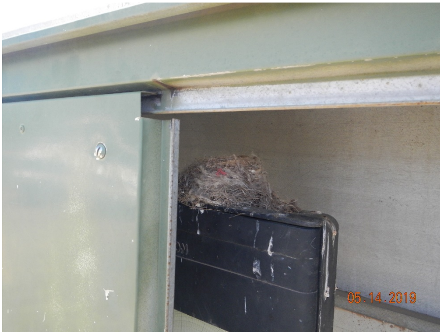
Active bird nest inside separator housing
