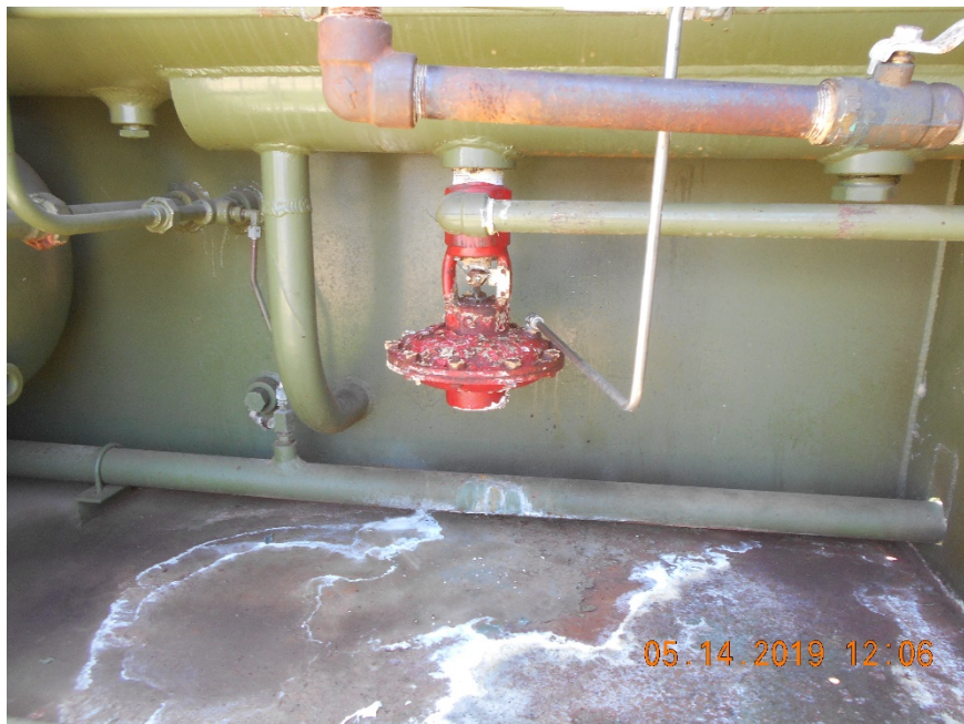
W side separator. Control valve with corrosion and staining.
