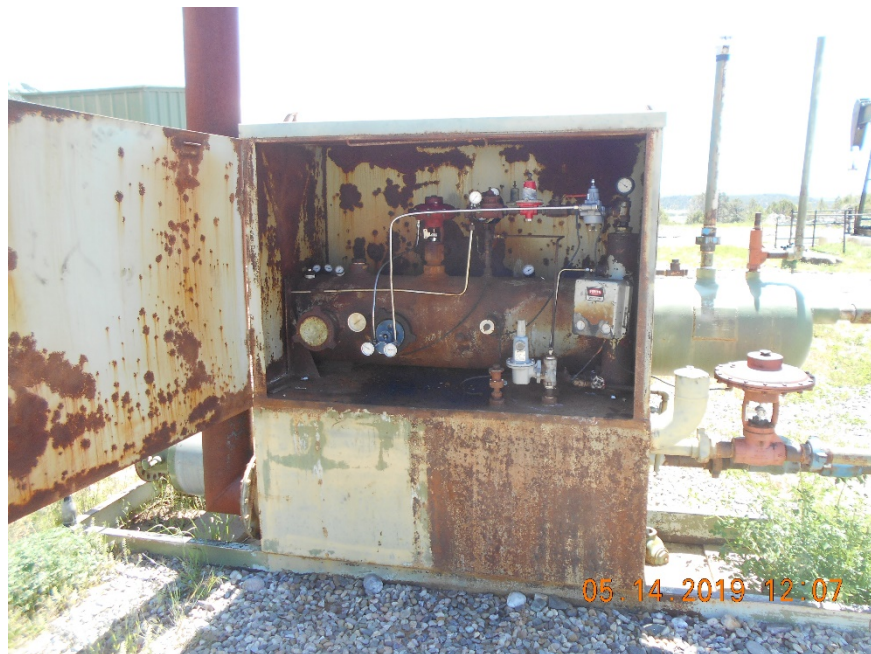
E side separator. Possible leaks detected. See FLIR photos for leak inspection.
