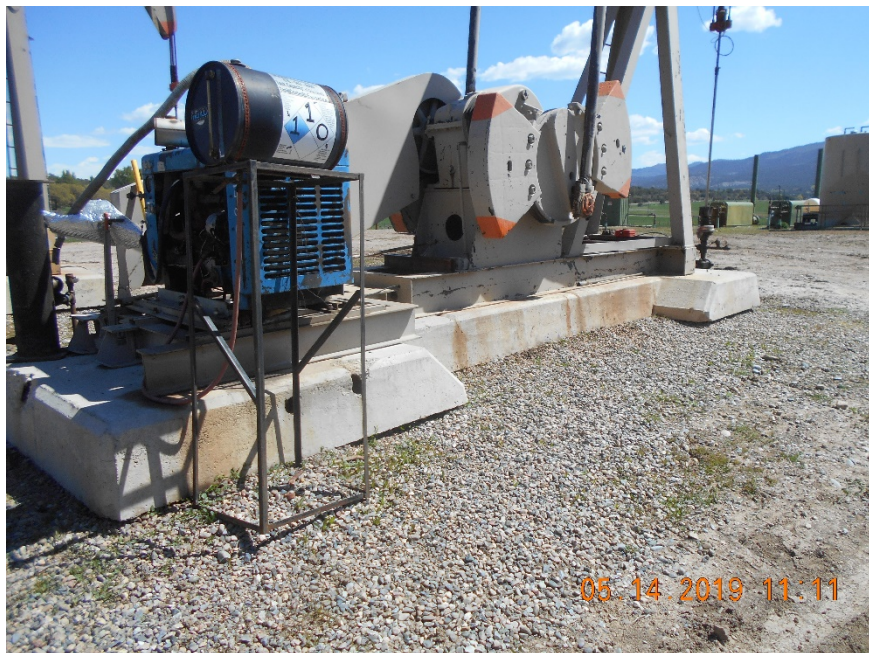
API # 05-067-09623 ARTFGANCE 33-7-14 #3C Motor oil container with no secondary containment
