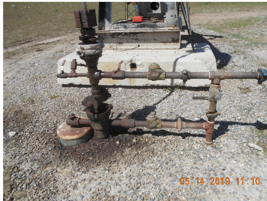
API # 05-067-09623 ARTFGANCE 33-7-14 #3C Wellhead with stained soil
