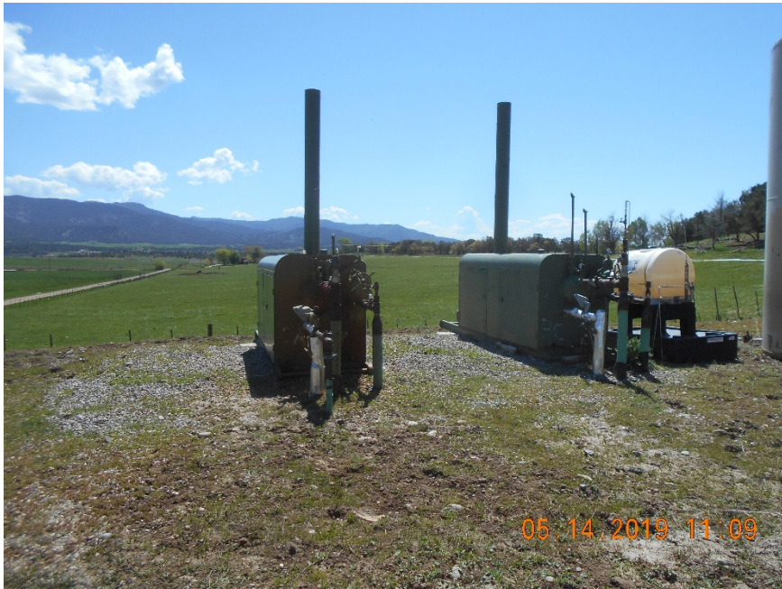
Separators with chemical injector in secondary containment
