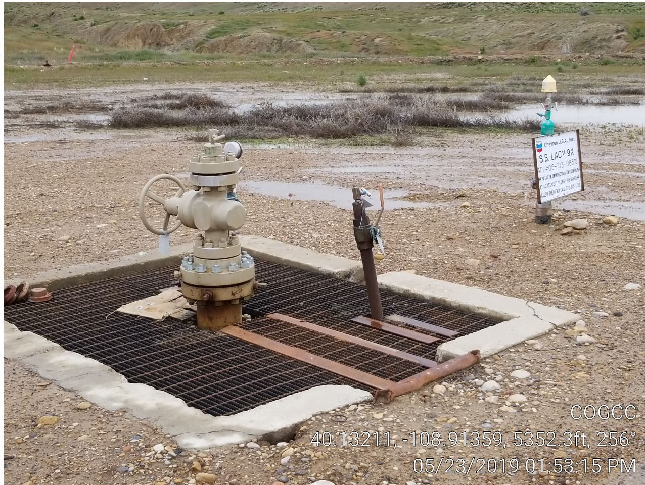
Photo 1. Location looking west.
