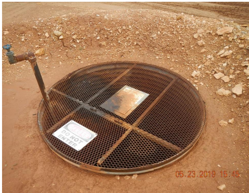
Open topped buried vessel labeled produced water.
