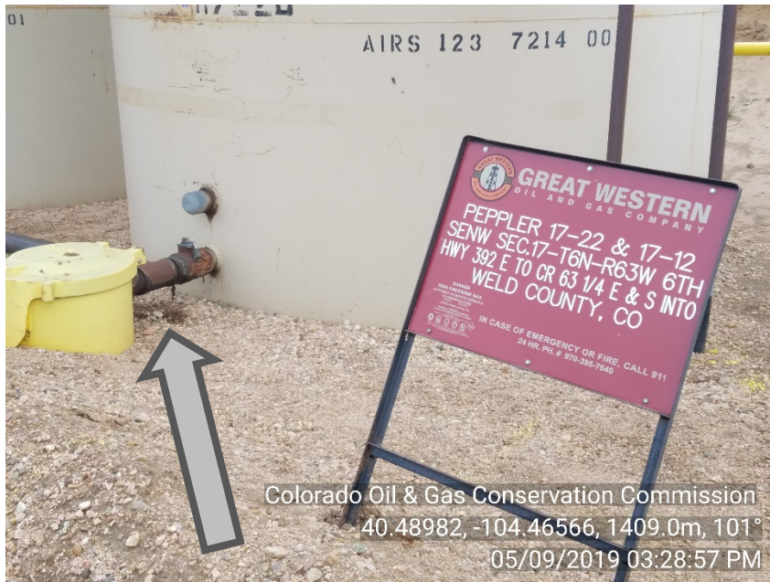
Photo #7 Peppler 17-12, 17-22 Battery West condensate tank - loadout Stained soil from prior insp.
