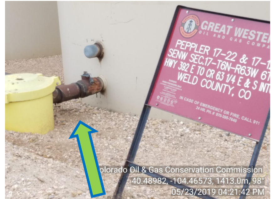
Photo #8 Peppler 17-12, 17-22 Battery West condensate tank - loadout Stained soil – Appears Mitigated
