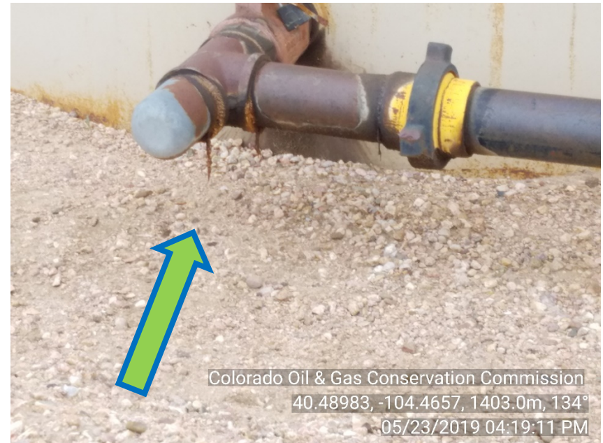
Photo #6 Peppler 17-12, 17-22 Battery East condensate tank - loadout Stained soil – Appears Mitigated
