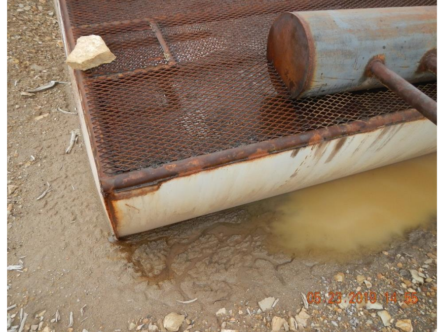
Stained soil in SE corner of vessel. Contents are overflowing.
