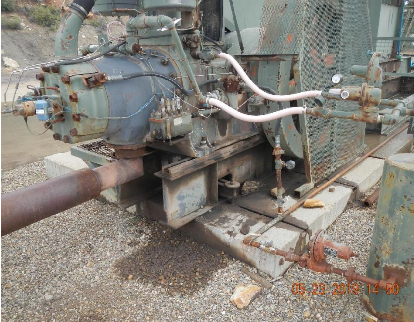
Concrete pad and gravel are stained beneath prime mover.
