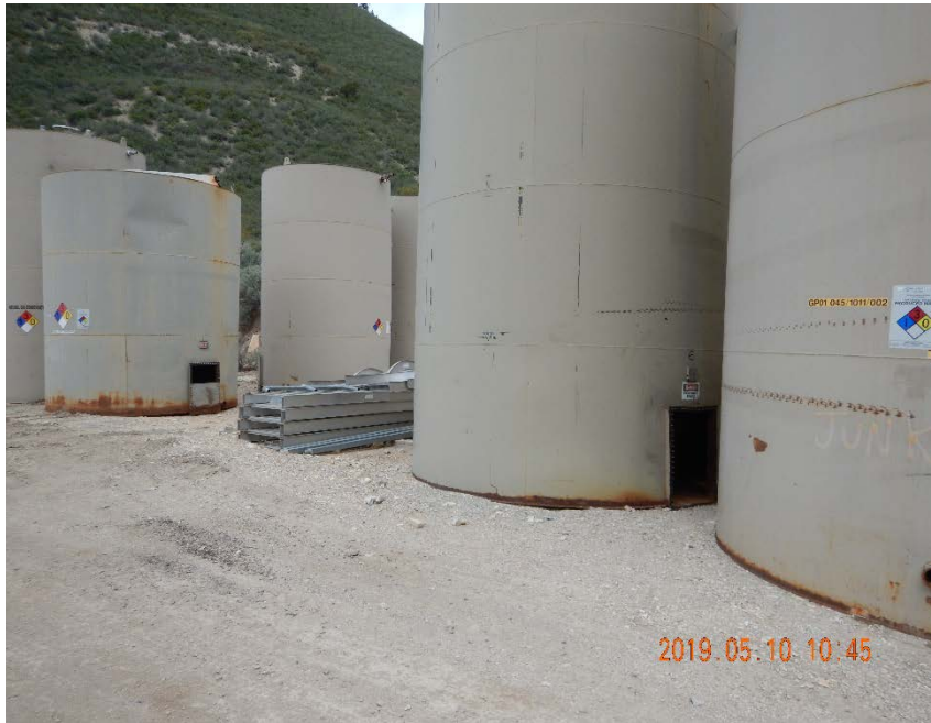
Photo #17 – View of unused tanks inside of storage area in NW corner of location. Note uncovered access panels on unused ASTs.
