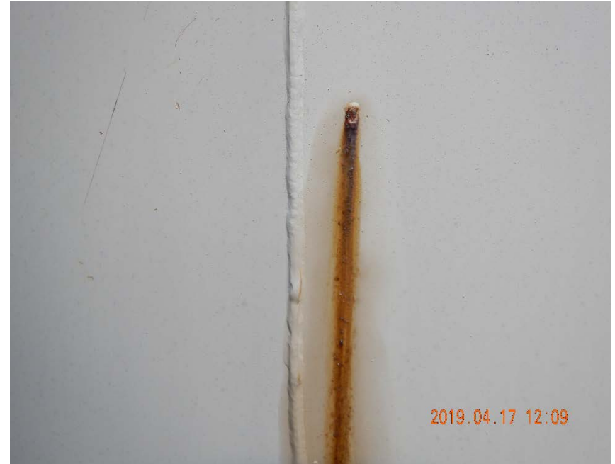
Photo #10 – Fluid and rust staining on southern crude oil AST. Operator was notified of potential fluid leak on 4/17/2019 via phone call. The suspect tank and tank battery were decommissioned and removed prior to 5/10/2019 follow-up inspection.
