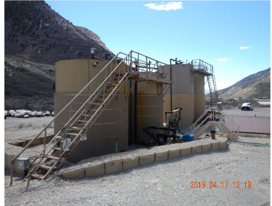
Photo #22 – View of truck loadout tank battery on east side of location, looking south. Note unlined secondary containment.
