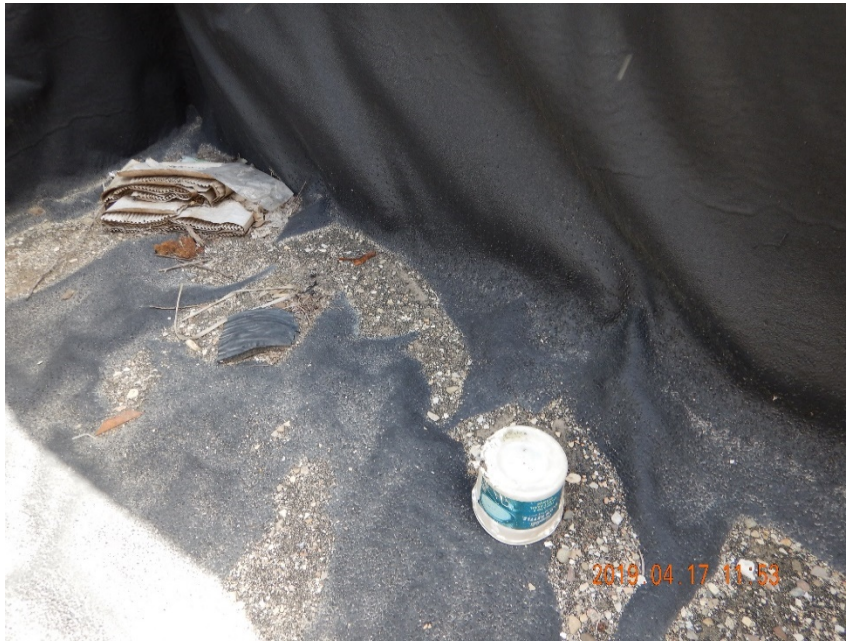
Photo #3 – Trash and wind-blown weeds accumulating inside of central tank battery secondary containment (1).
