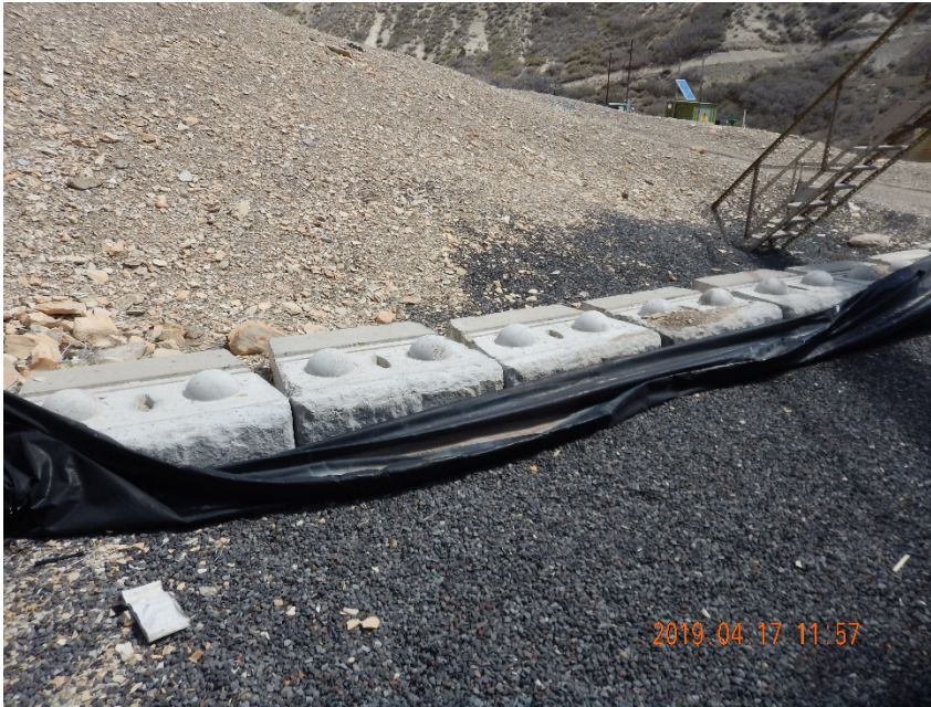
Photo #5 - View of tank battery liner NE of 500 bbl produced water/condensate AST. Note that liner is not secured along wall.
