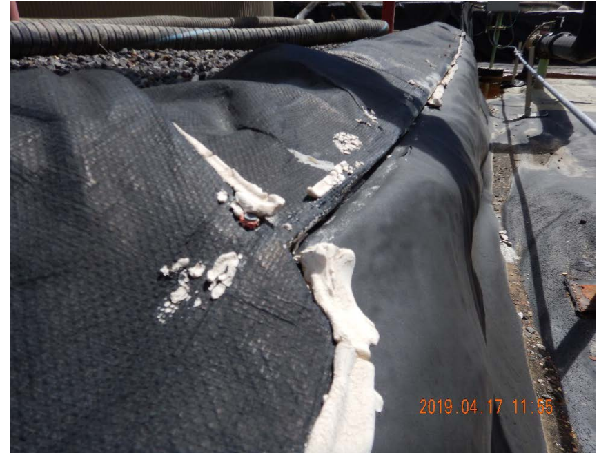
Photo #6 – View of liner seam between 500 bbl produced water/condensate AST battery from previous photo and central tank battery. Liner and seam in disrepair. Note liner is secured and punctured with nails in this area.
