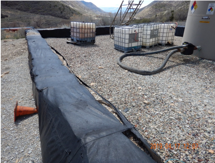
Photo #9 - View of shredded tank liner, looking south. Several holes in liner were observed on 4/17/2019 inspection date.
