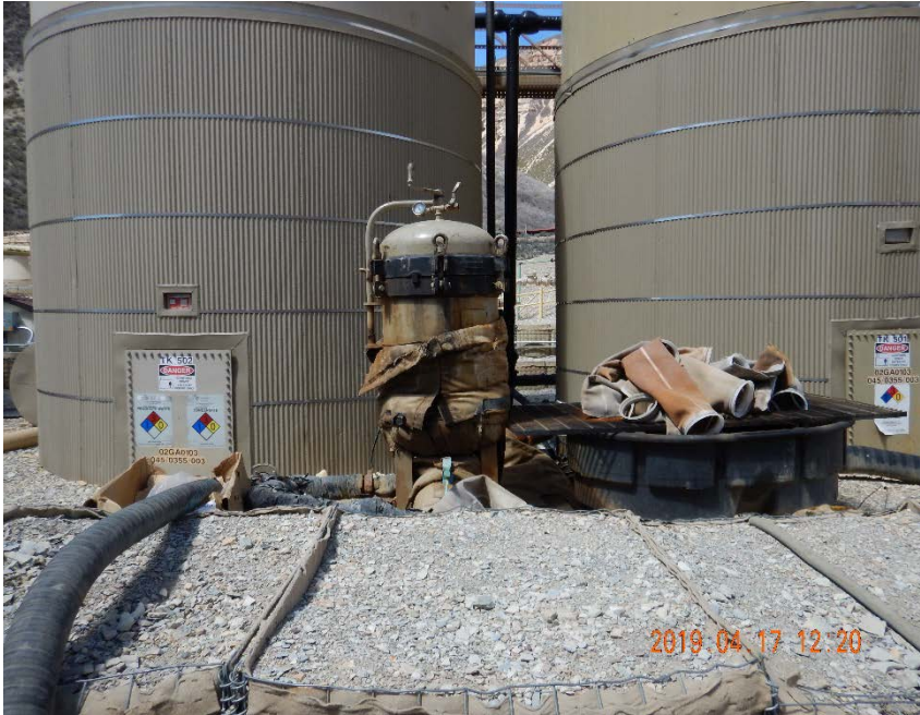
Photo #25 – View of filter pot on east side of truck loadout tank battery. Note storage of filter socks atop secondary containment device.
