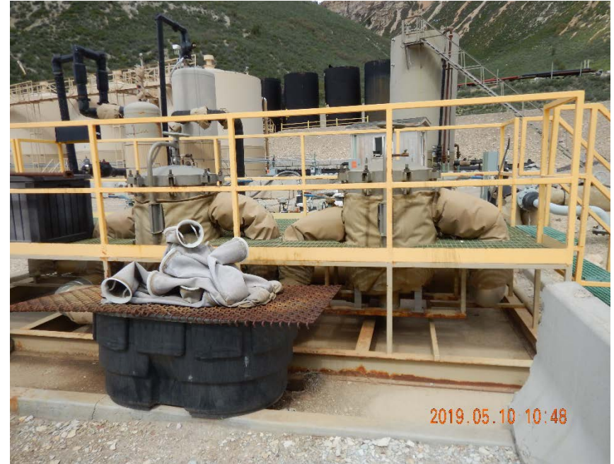
Photo #20 – View of filter pots and filter socks, looking west. Note storage of filter socks atop secondary containment device.
