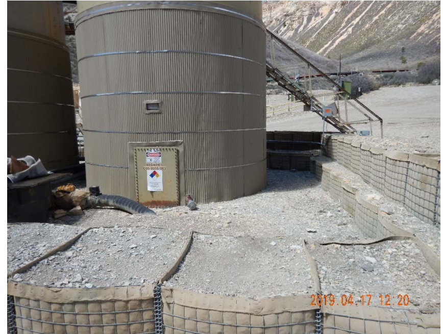
Photo #24 – View of north side of truck loadout tank battery, looking west. Note berm is constructed of unconsolidated material inside of canvas and mesh crates. Secondary containment area did not have a liner installed on either inspection date.
