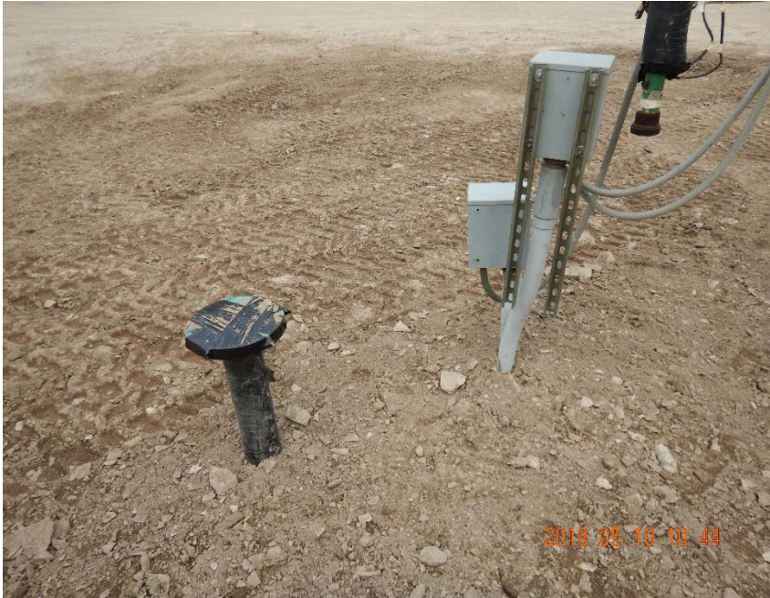
Photo #15 – Unmarked, unused flowline riser near wellhead.
