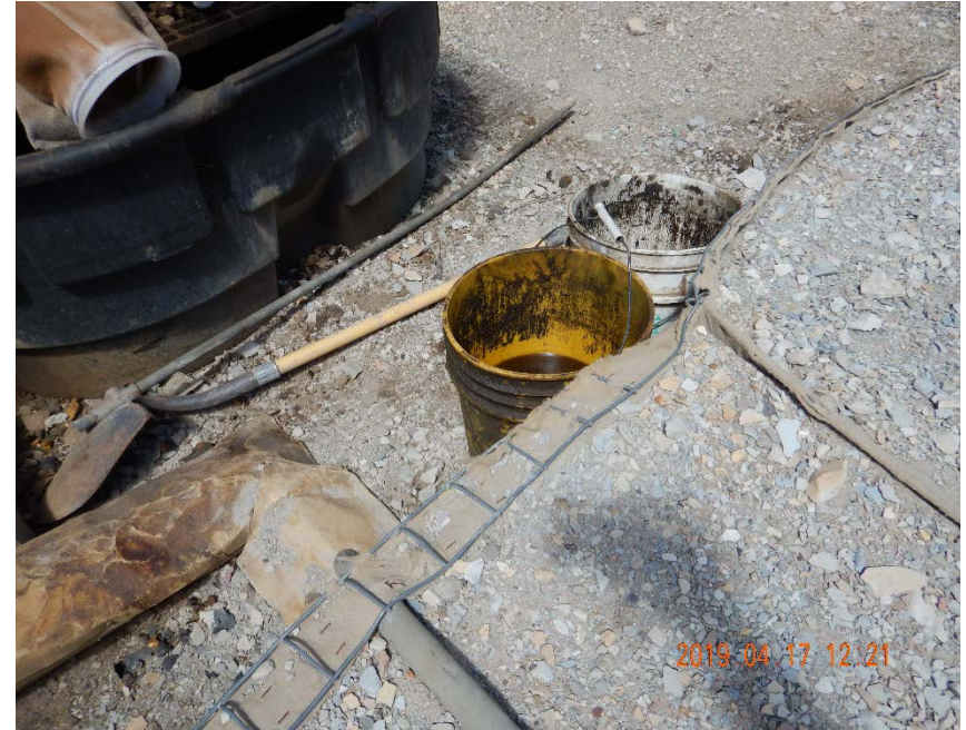
Photo #26 – Uncovered buckets of oily fluid stored inside of truck loadout tank battery.
