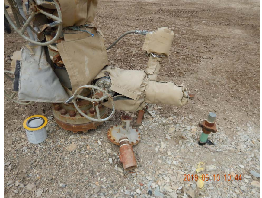
Photo #16 – Unmarked, unused flowline riser with bullplug near wellhead.
