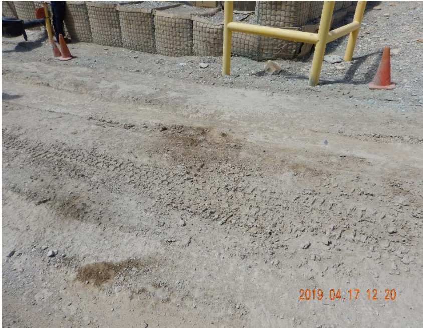
Photo #23 – Localized accumulations of oil-stained soil and truck ruts located NE of truck loadout tank battery. Operator should consider a concrete apron or liner system at the truck loadout.
