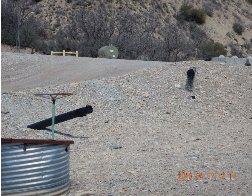
Photo #21 – View of unmarked HDPE flowlines located ~70' NE of central tank battery.
