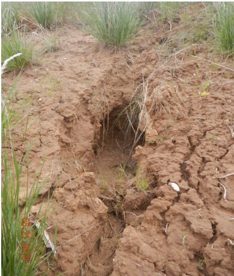
Photo#5: Erosion on Cut Slope.
