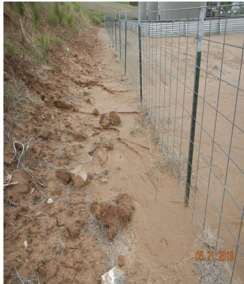
Photo#6: Sediment migrating from Cut slope.
