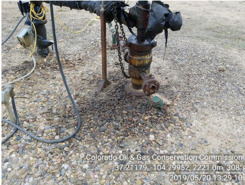
PHOTO 3: AREA OF IMPACTED SOIL APPROX. 3' x 2' NEAR WELLHEAD. Securely fasten all valves, pipes, and fittings to ensure good mechanical condition, inspect at regular intervals and maintain in good mechanical condition per Rule 605.d. Non E&P Waste not properly stored, handled, transported, treated, or disposed per Rule 907A. CA DATE 6/20/19
