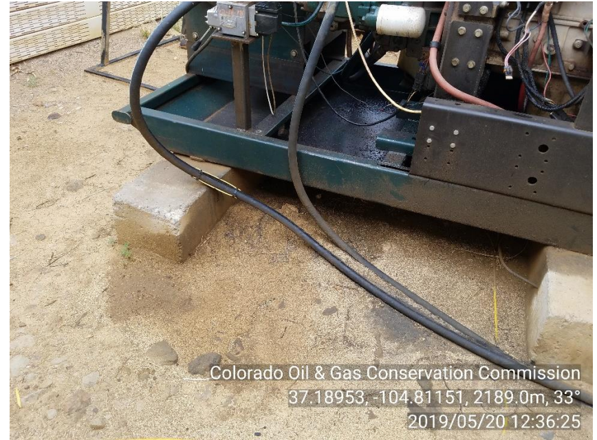
PHOTO 4: Engine skid stained soil around skid. Securely fasten all valves, pipes, and fittings to ensure good mechanical condition, inspect at regular intervals and maintain in good mechanical condition per Rule 605.d. Remove or remediate stained soil. Ca date 6/20/19
