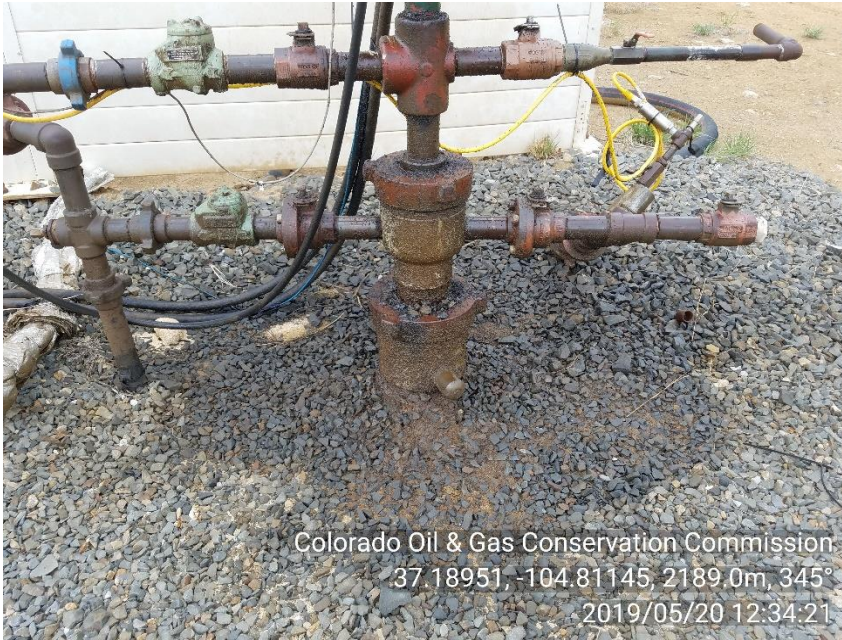
PHOTO 3: Hydraulic Stained soil at base of wellhead approx 6'x 3'. Securely fasten all valves, pipes, and fittings to ensure good mechanical condition, inspect at regular intervals and maintain in good mechanical condition per Rule 605.d. Remove or remediate stained soil. Ca date 6/20/19
