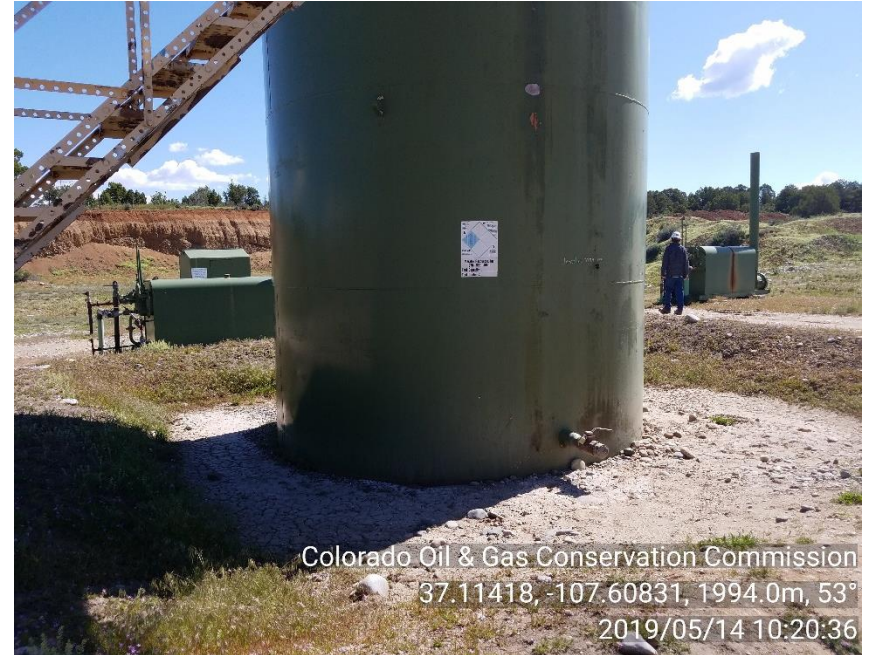
PHOTO 2: TANK BATTERY/ NFPA STICKER IS FADED AND IS NOT LEGIBLE. Install sign to comply with Rule 210. CA DATE 6/21/19
