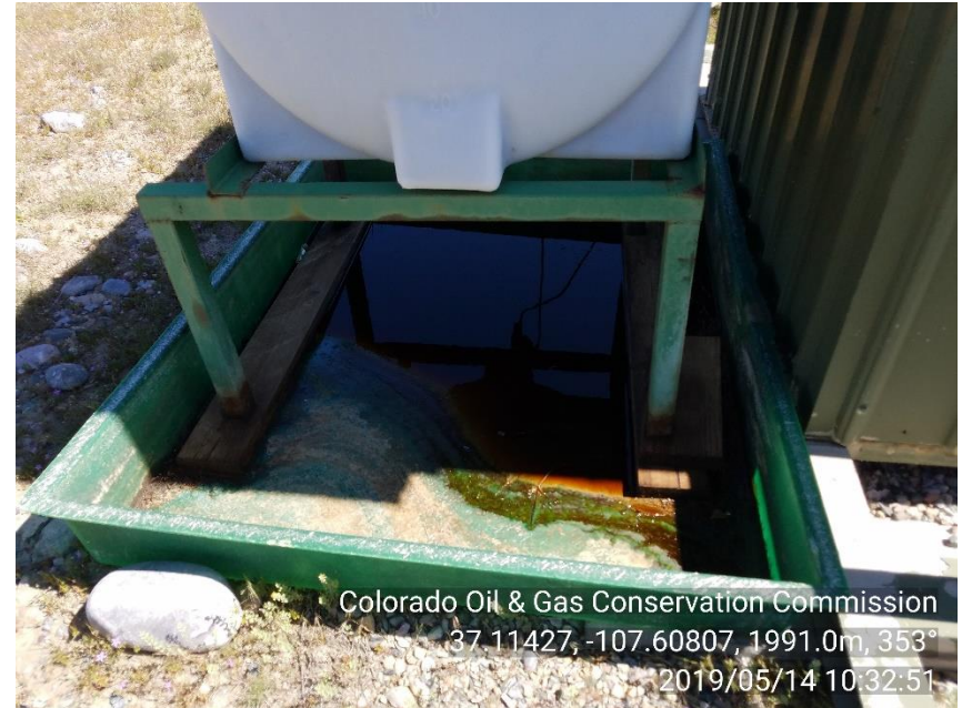
PHOTO 12: There is a dark oily fluid in the spill prevention by the meter house. Comply with SB-181 and general provisions of the oil and gas act for wildlife protection. CA date 5/21/19.
