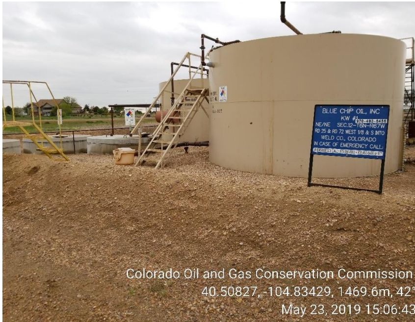
Photo 1: Centralized Tank Battery
