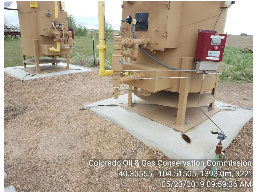
ECD anchoring on 5/23/19
